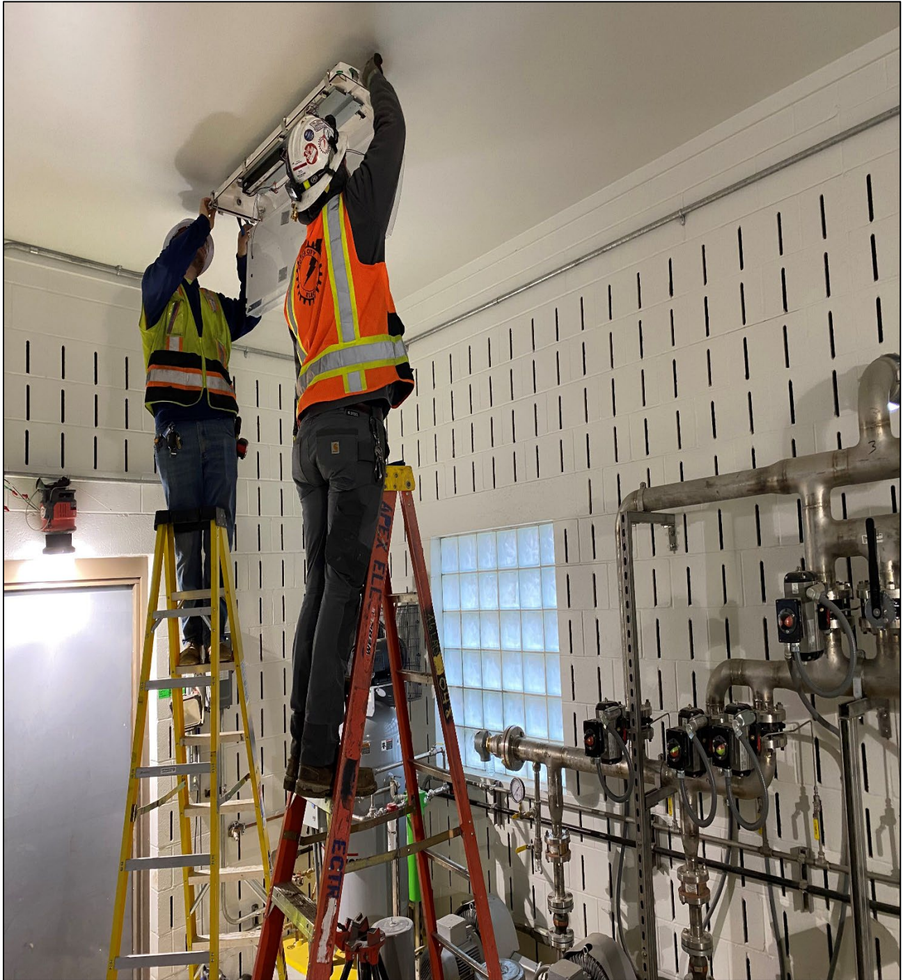
Figure 8 – Installing New Lighting at Beaconsfield Control Bldg.
