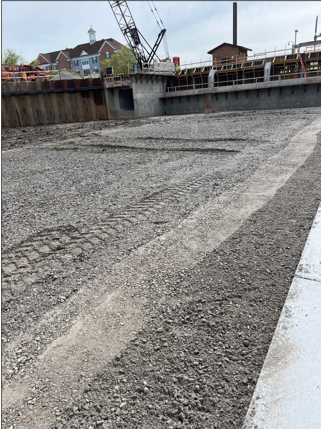
Figure 21 – Canal Bottom Excavation (exposing finished face of sheeting)
