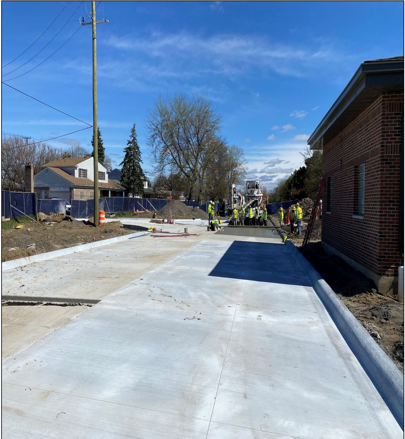
Figure 7 – Pouring Beaconsfield Road Concrete
