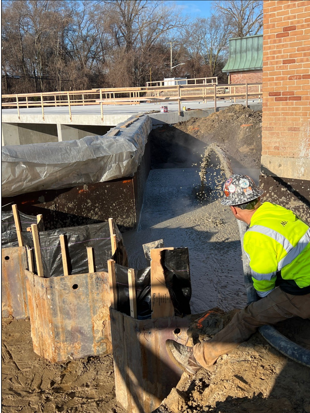
Figure 26 – Lightweight Concrete Pour south of Aeration Building
