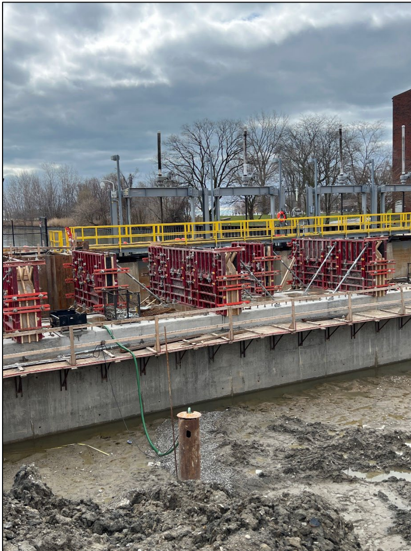
Figure 15 – Divider Wall Forms
