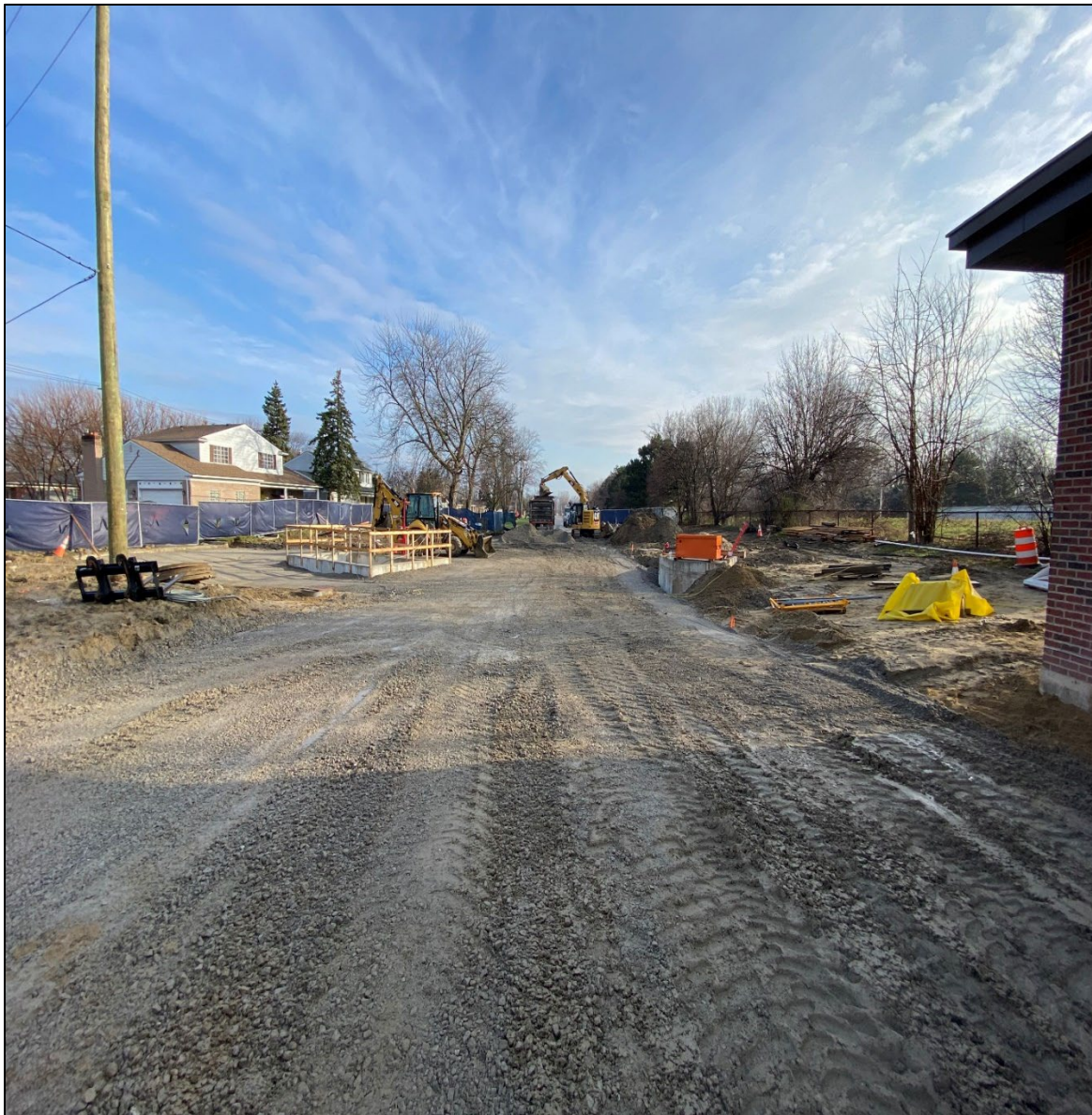
Figure 1 – Placing Stone Sub-Base for Concrete Pavements @ Beaconsfield Rd.
