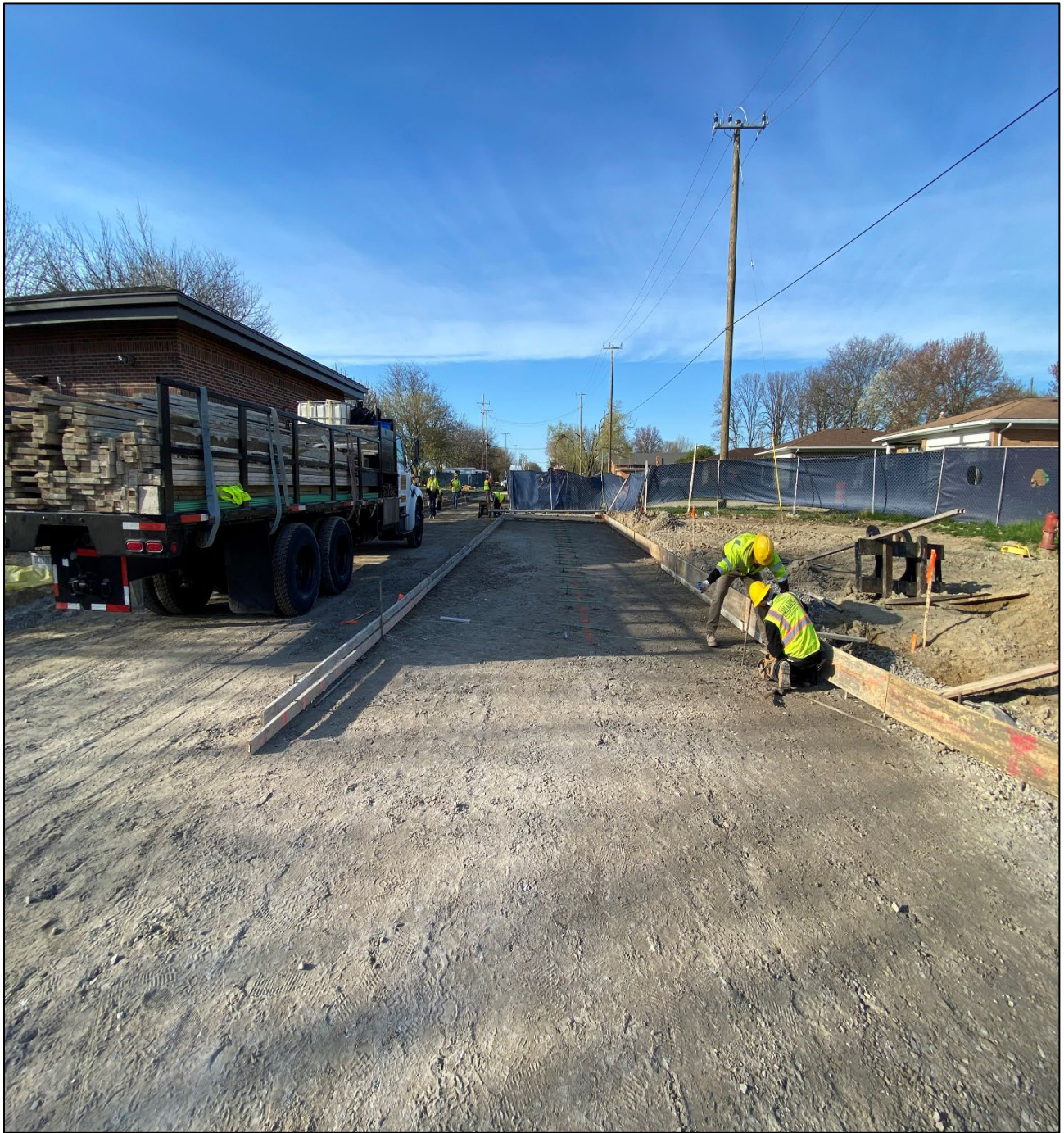
Figure 4 – Setting Forms for New Concrete @ Beaconsfield Site
