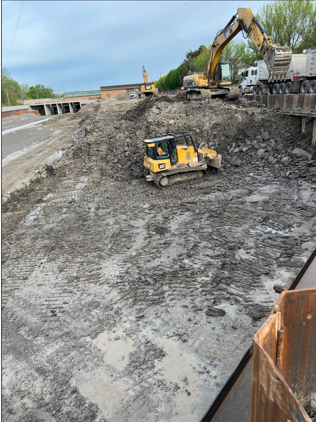
Figure 20 – Canal Bottom Excavation (exposing finished face of sheeting)
