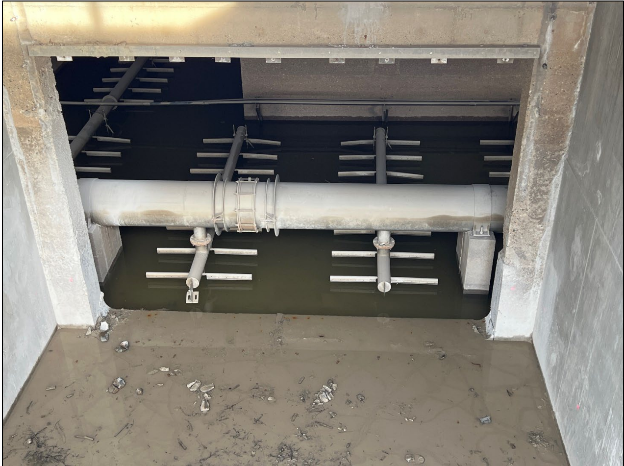
Figure 25 – Aeration Chamber Outfall - Screens/Wall removed for enlarged opening from RTB
