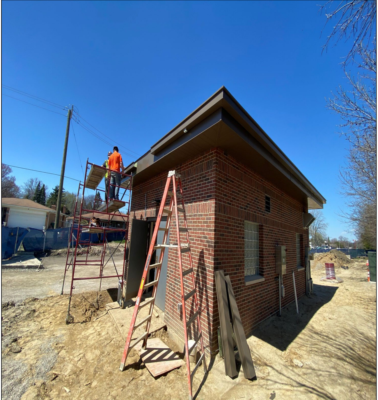
Figure 11 – Hanging Gutters & Downspouts @ Beaconsfield Control Building
