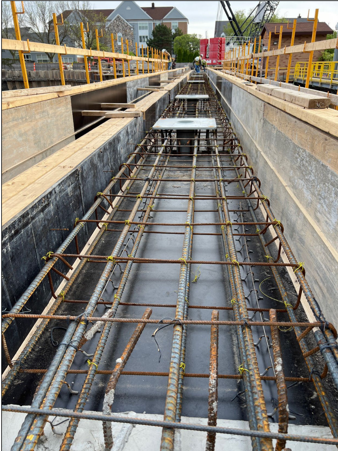
Figure 19 – Top Slab Rebar and embedded Davit Crane bases
