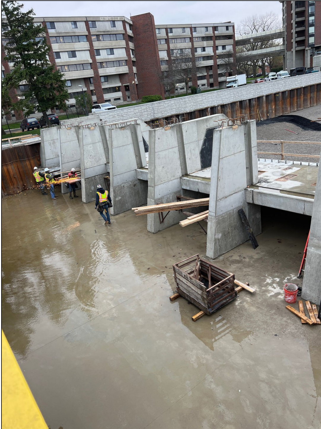
Figure 17 – Divider Walls Completed
