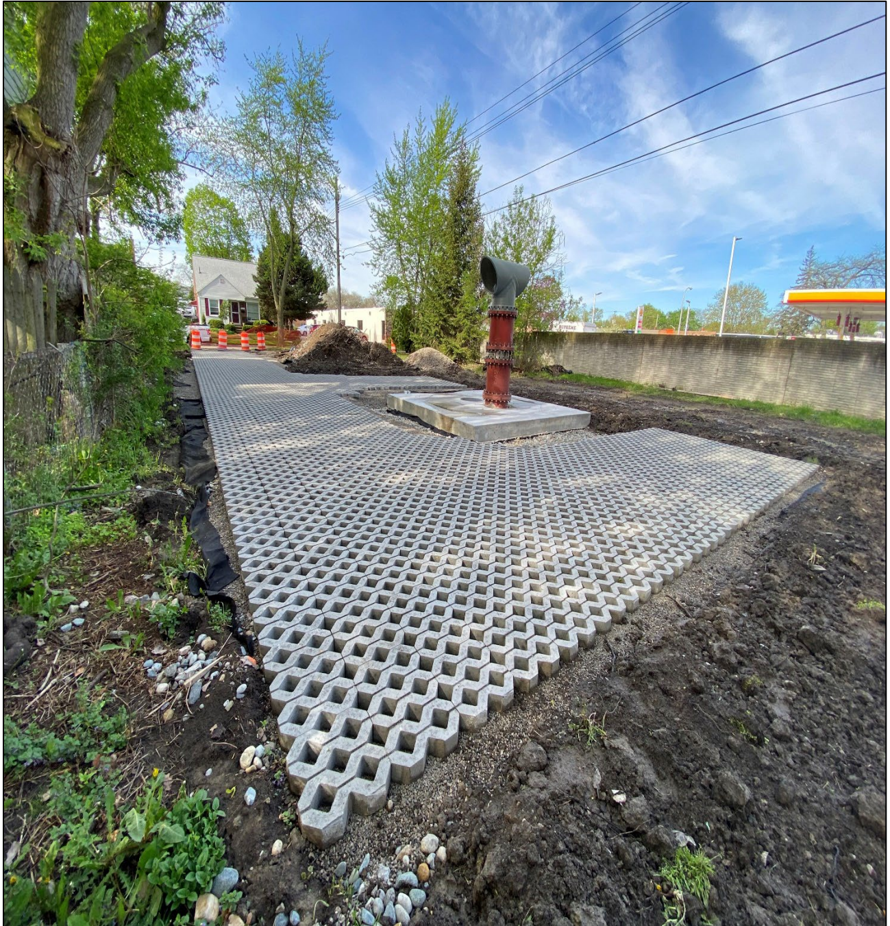
Figure 13 – Placing Pavers for Gaukler Site Access Driveway
