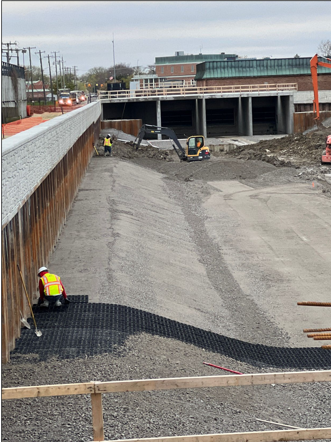
Figure 22 – Canal Bottom & Buttress - Grading, Stone, Geogrid, and Stone installation
