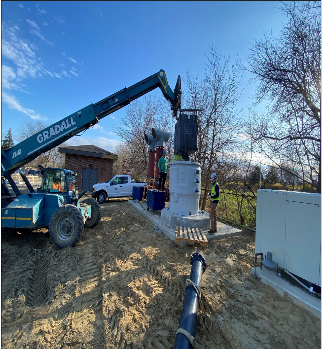
Figure 10 – Filling Odor Control Canister w/ Carbon Media @ Beaconsfield Site
