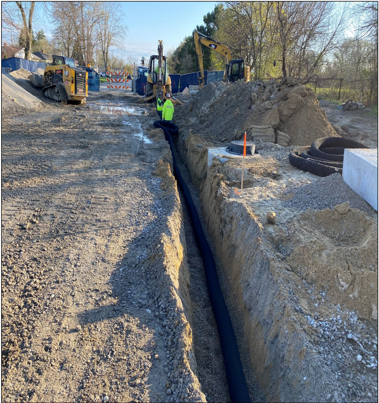
Figure 3 – Installing Underdrain under Pavements @ Beaconsfield Site
