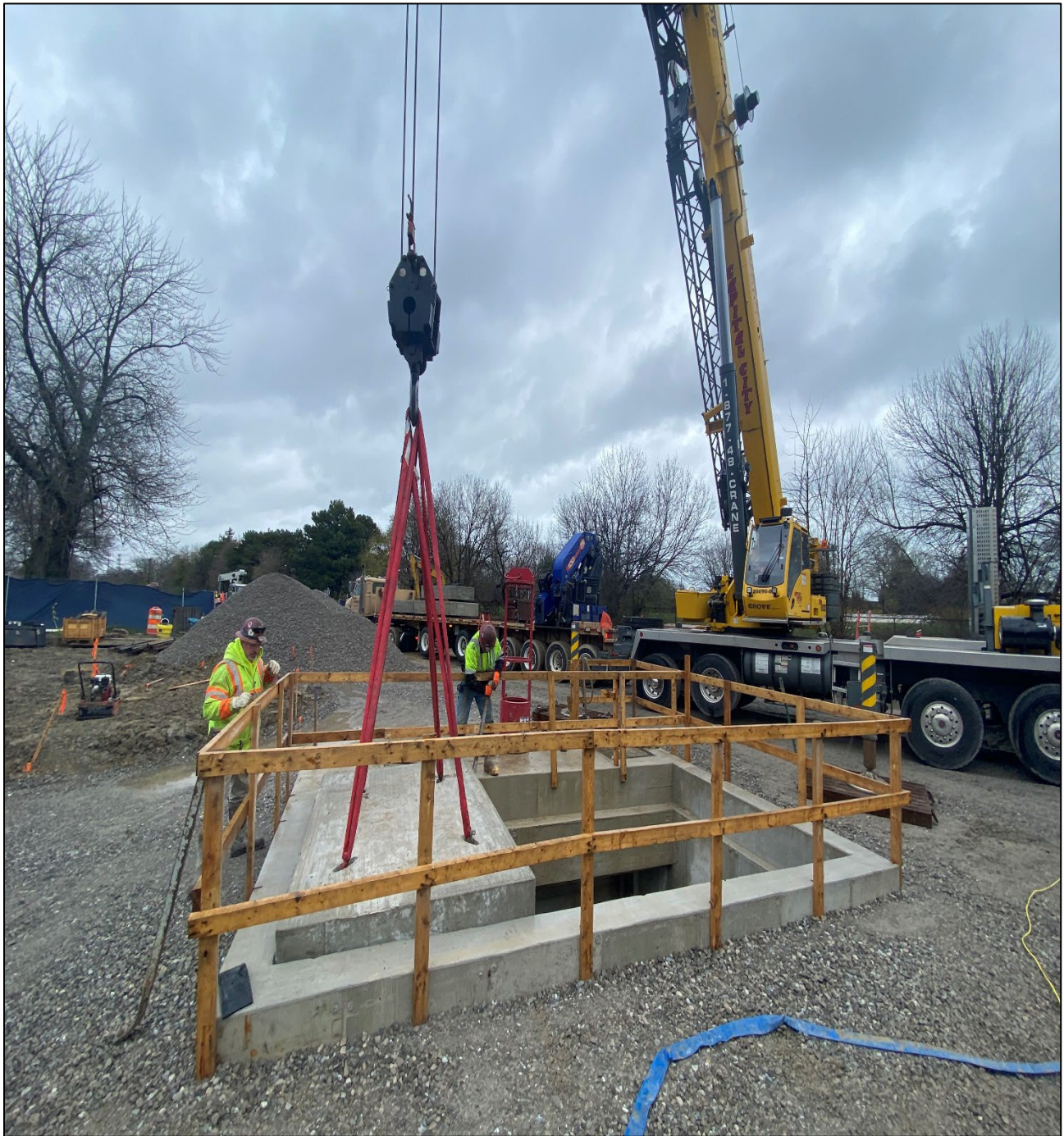
Figure 5 – Placing Precast Panel Over Access Vault @ Beaconsfield Site
