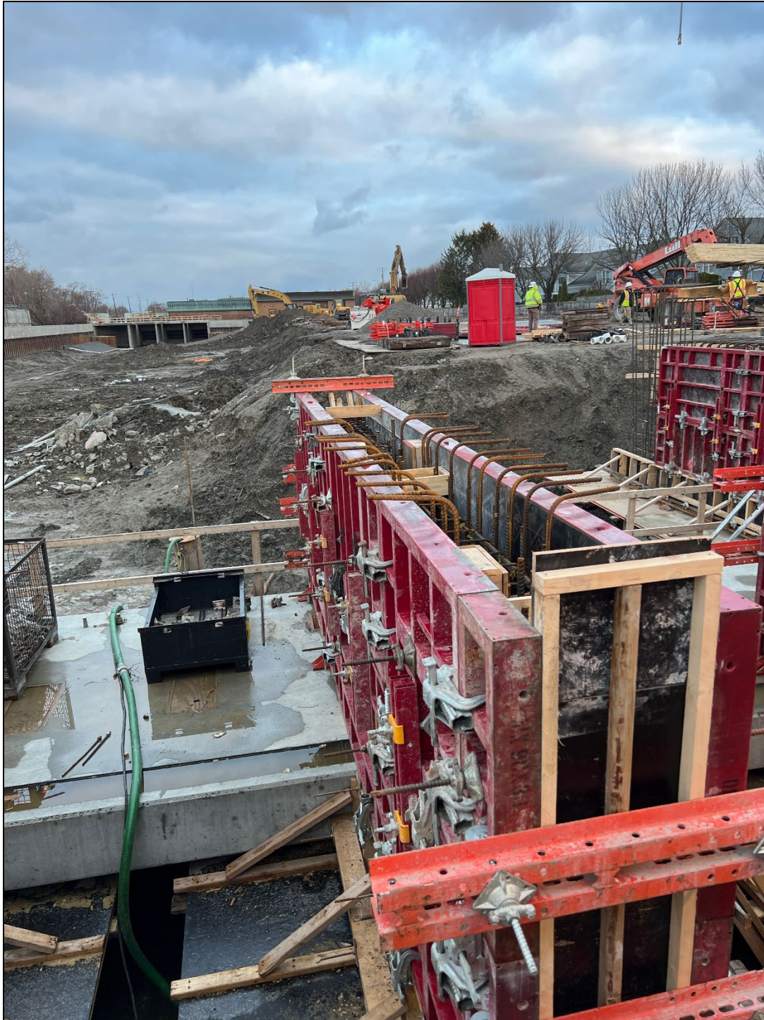
Figure 16 – Divider Wall Forms & Rebar
