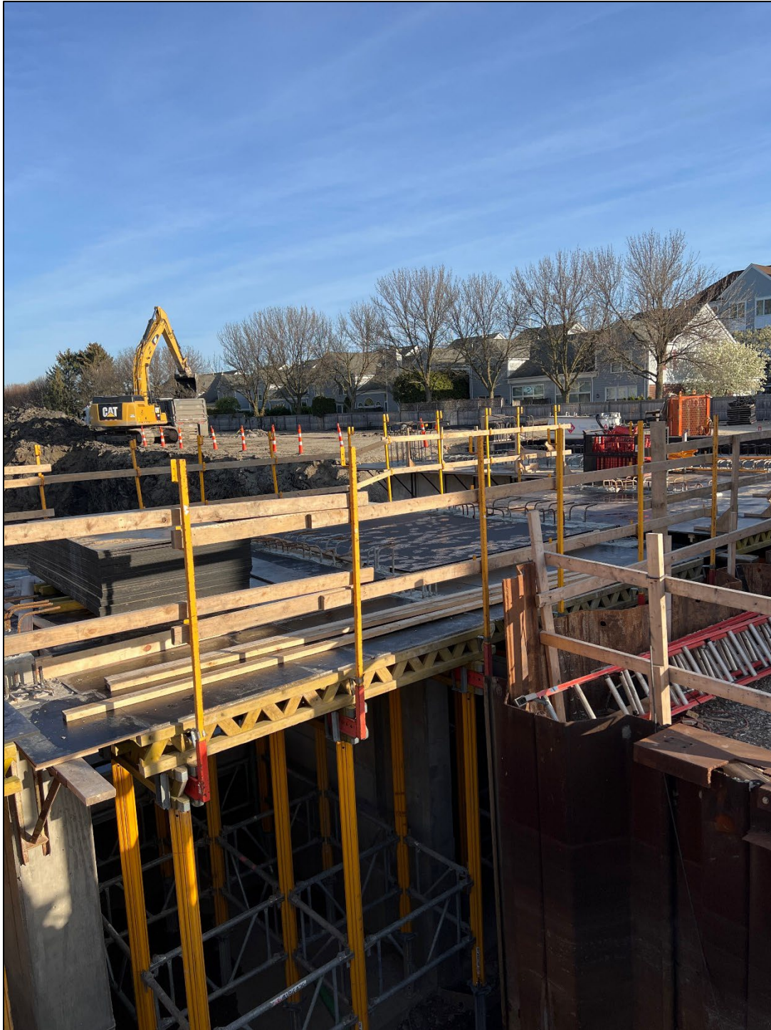
Figure 18 – Top Slab Forms
