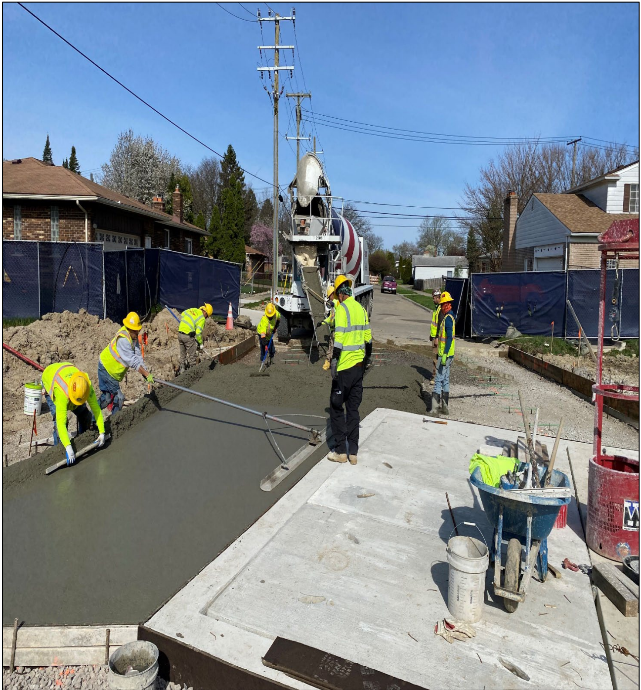
Figure 6 – Pouring Concrete at Beaconsfield & Oak Intersection
