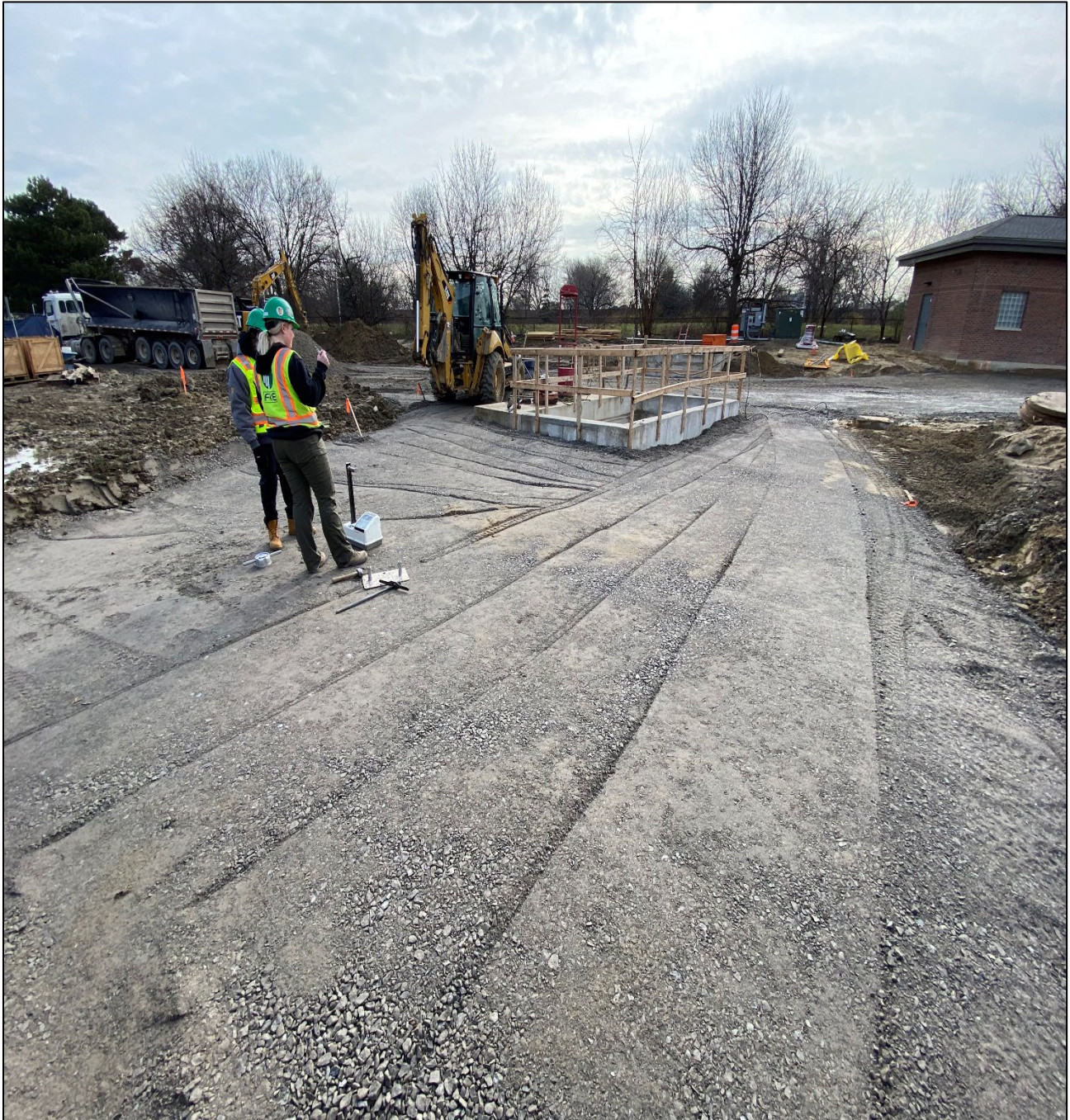
Figure 2 – Testing Stone Sub-Base Compaction @ Beaconsfield Site
