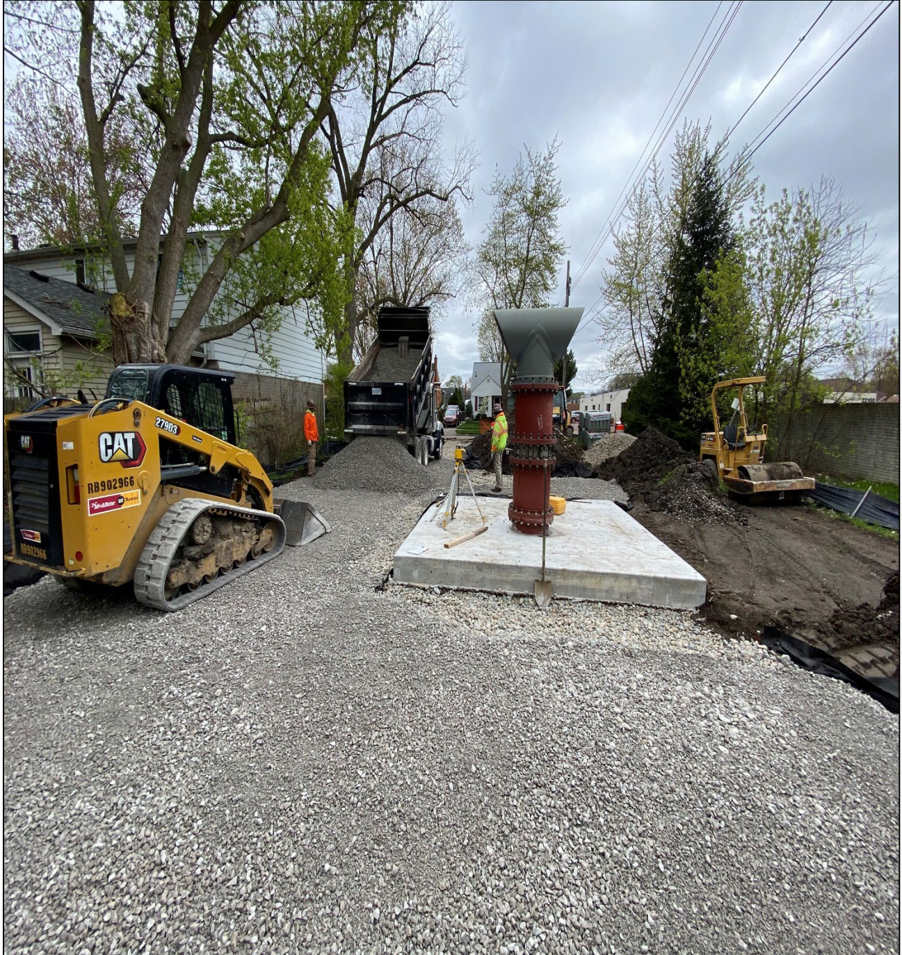
Figure 12 – Placing Stone Sub-Base for Gaukler Site Access Driveway
