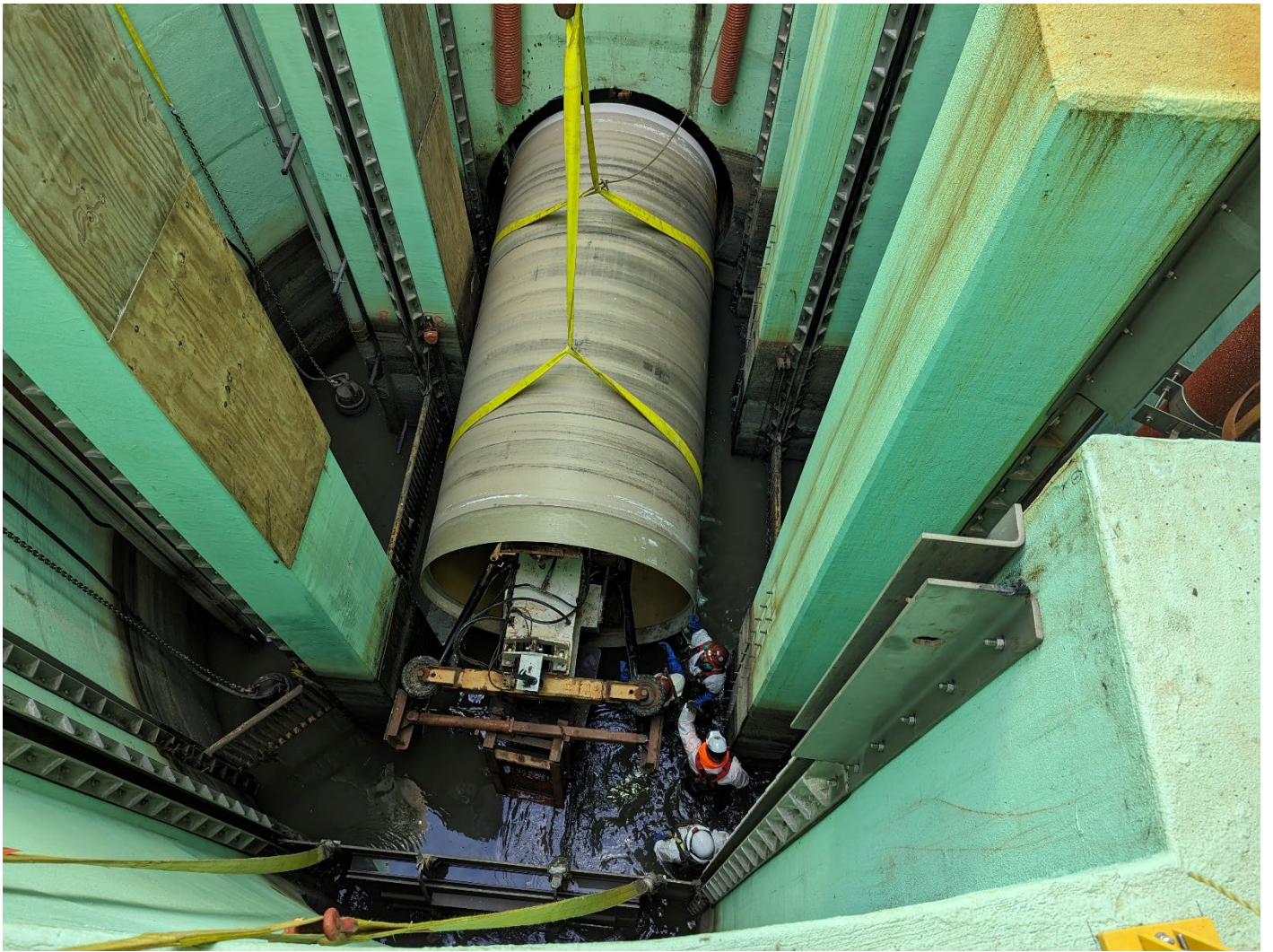
Figure 2 – Pipe Carrier Testing with HOBAS
