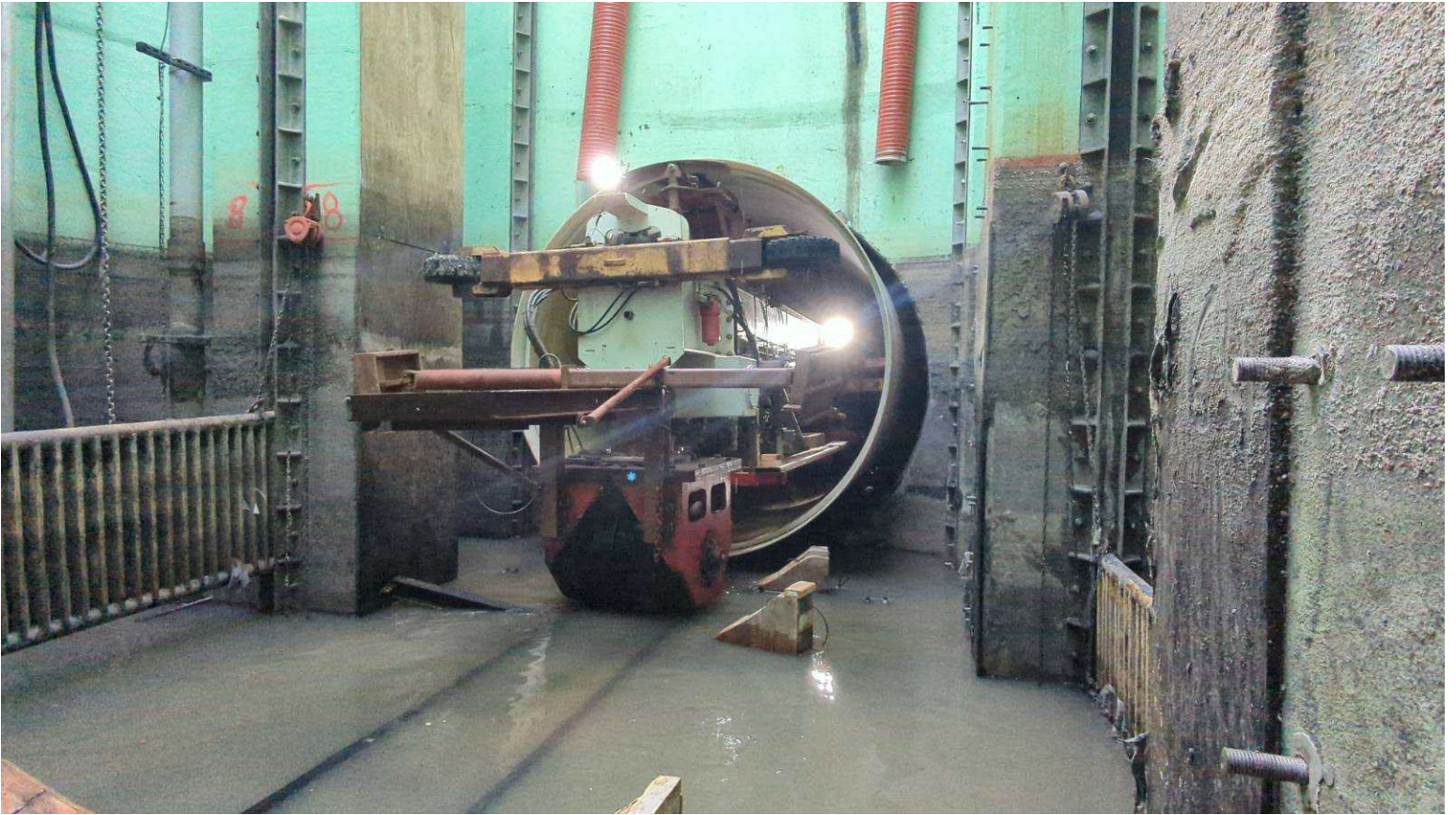
Figure 4 – Pipe Carrier Testing with HOBAS
