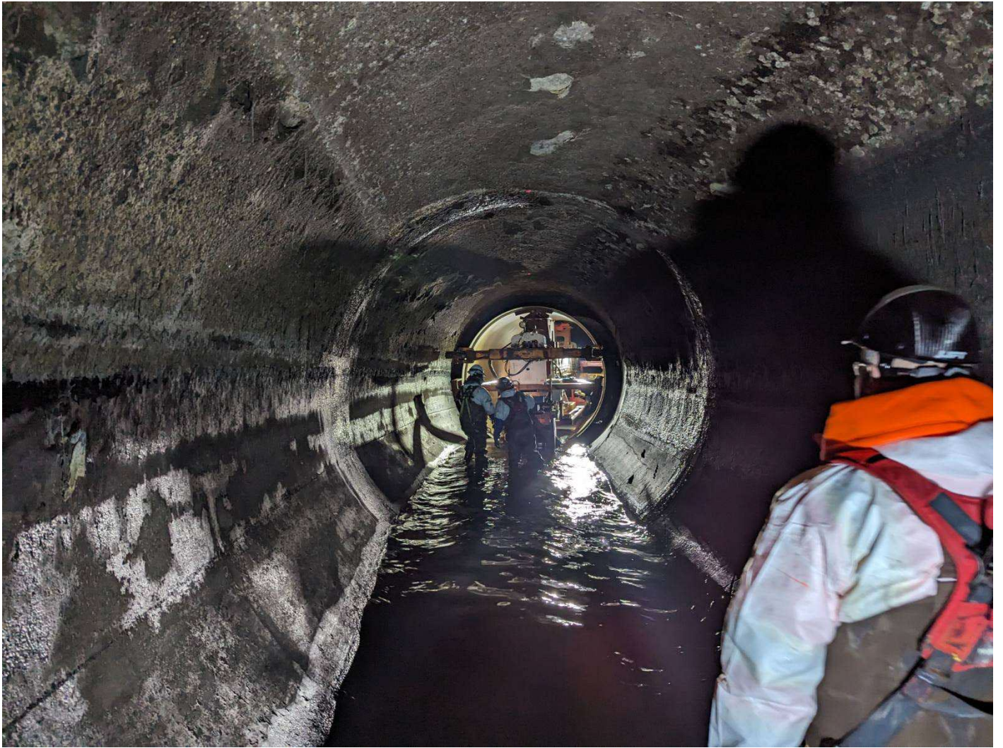
Figure 6 – Pipe Carrier Testing with HOBAS
