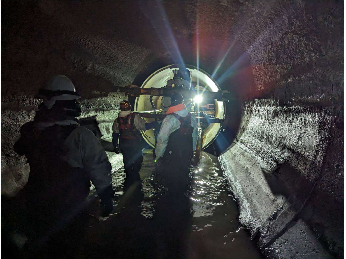
Figure 5 – Pipe Carrier Testing with HOBAS Pipe
