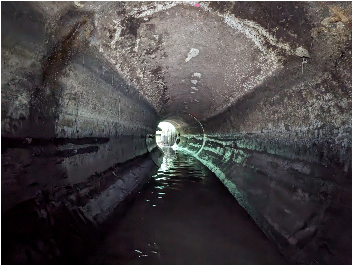
Figure 8 – RAI Curve Facing CS-12
