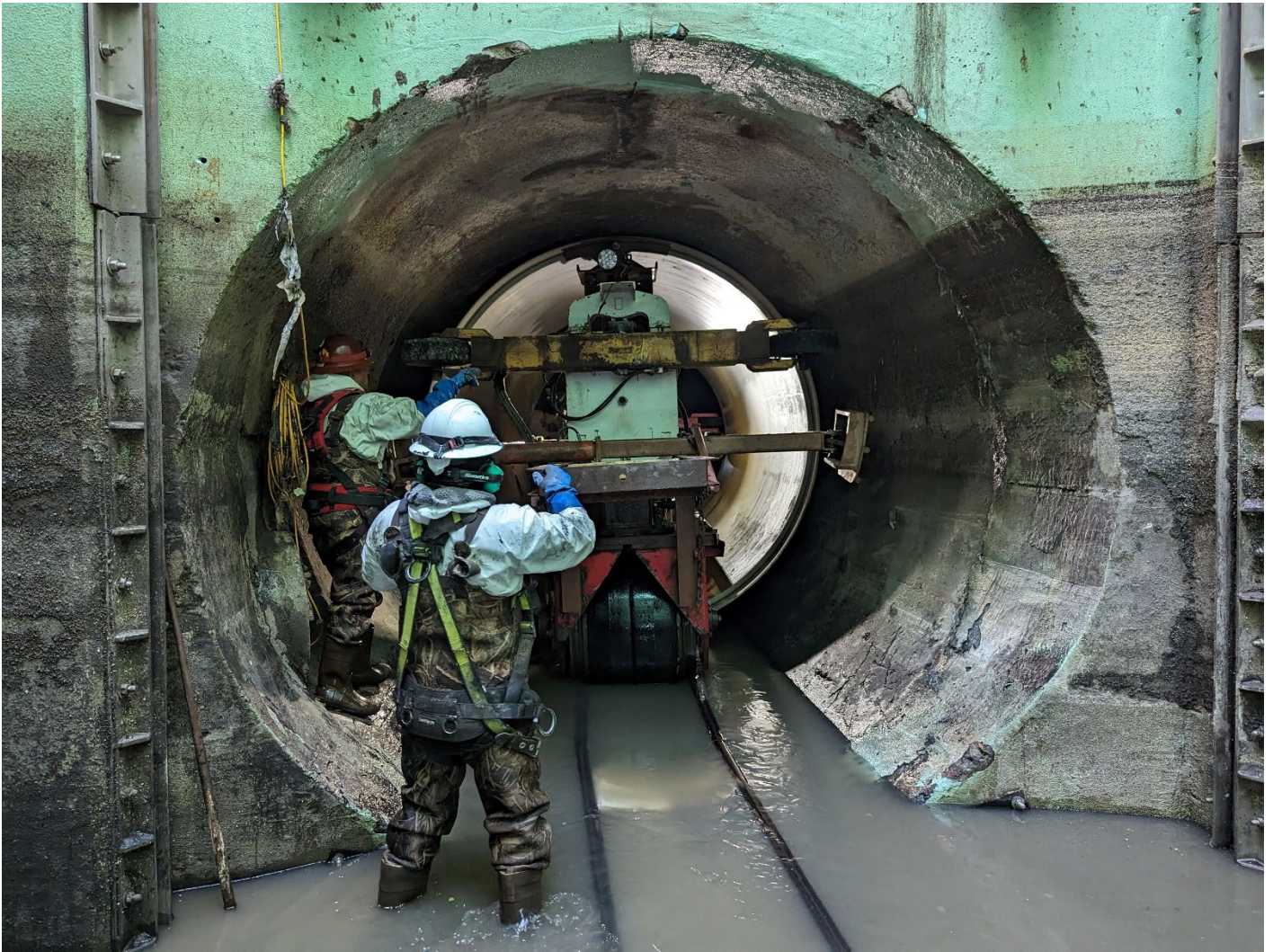
Figure 7 – Pipe Carrier Testing with HOBAS
