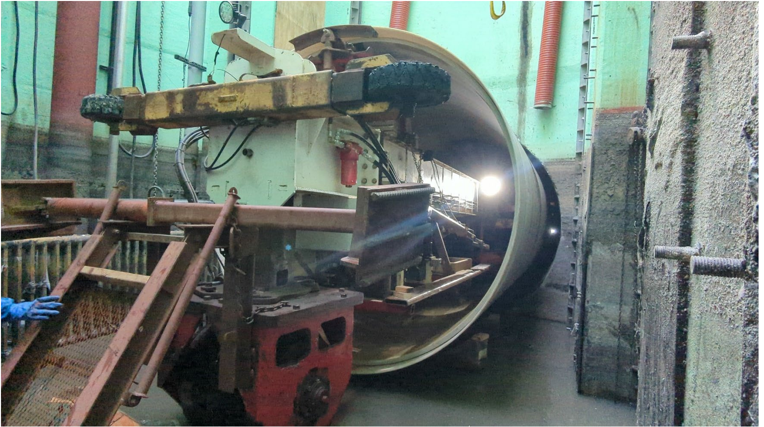
Figure 3 – Pipe Carrier Testing with HOBAS
