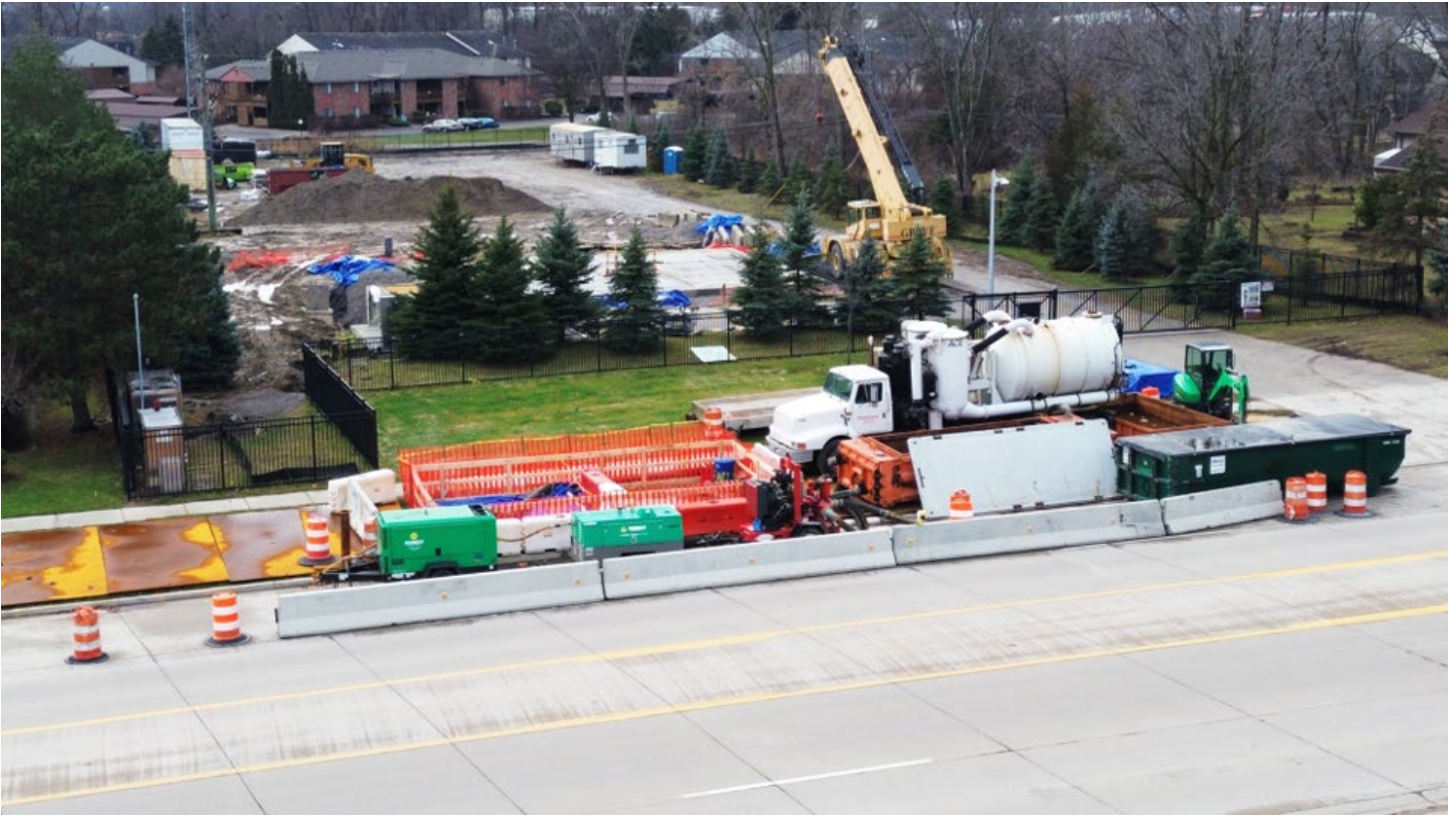
Figure 9 – Aerial View at CS-3 of Debris Removal Equipment
