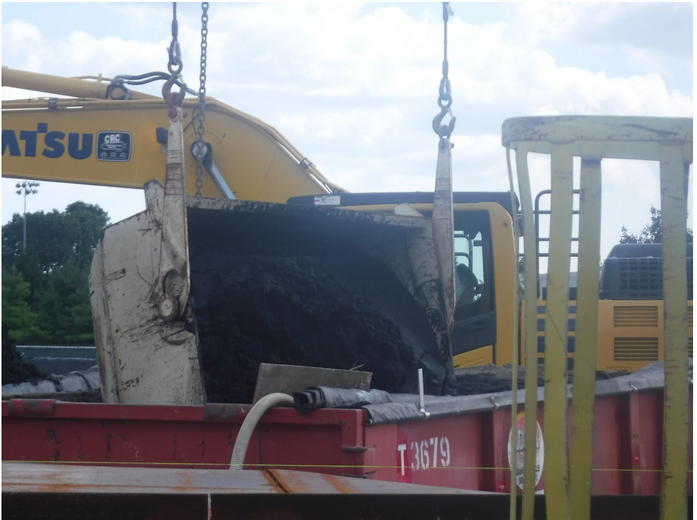
Figure 2 – Unloading Debris at CS-12
