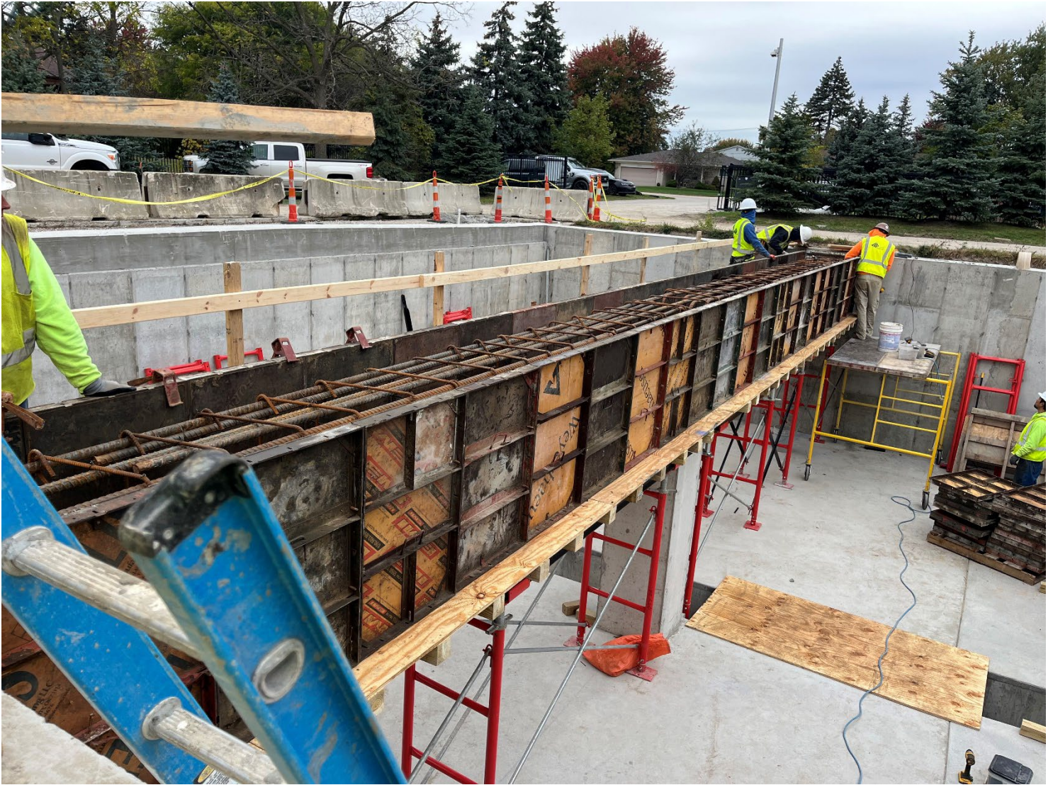
Figure 13 – Fraser Bio-Filter Roof Beam Construction
