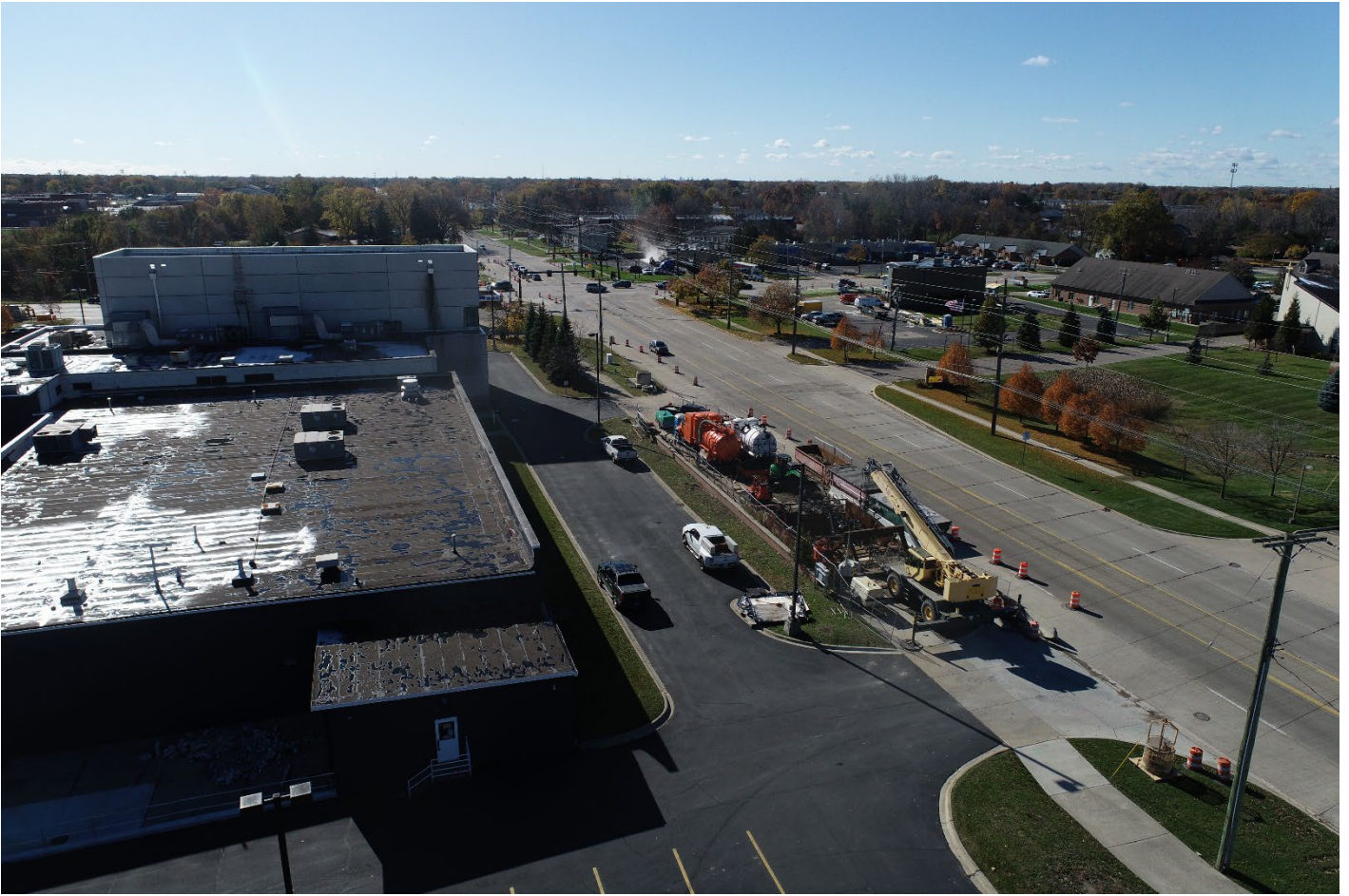
Figure 7 – Aerial View at CS-2 of Debris Removal Equipment
