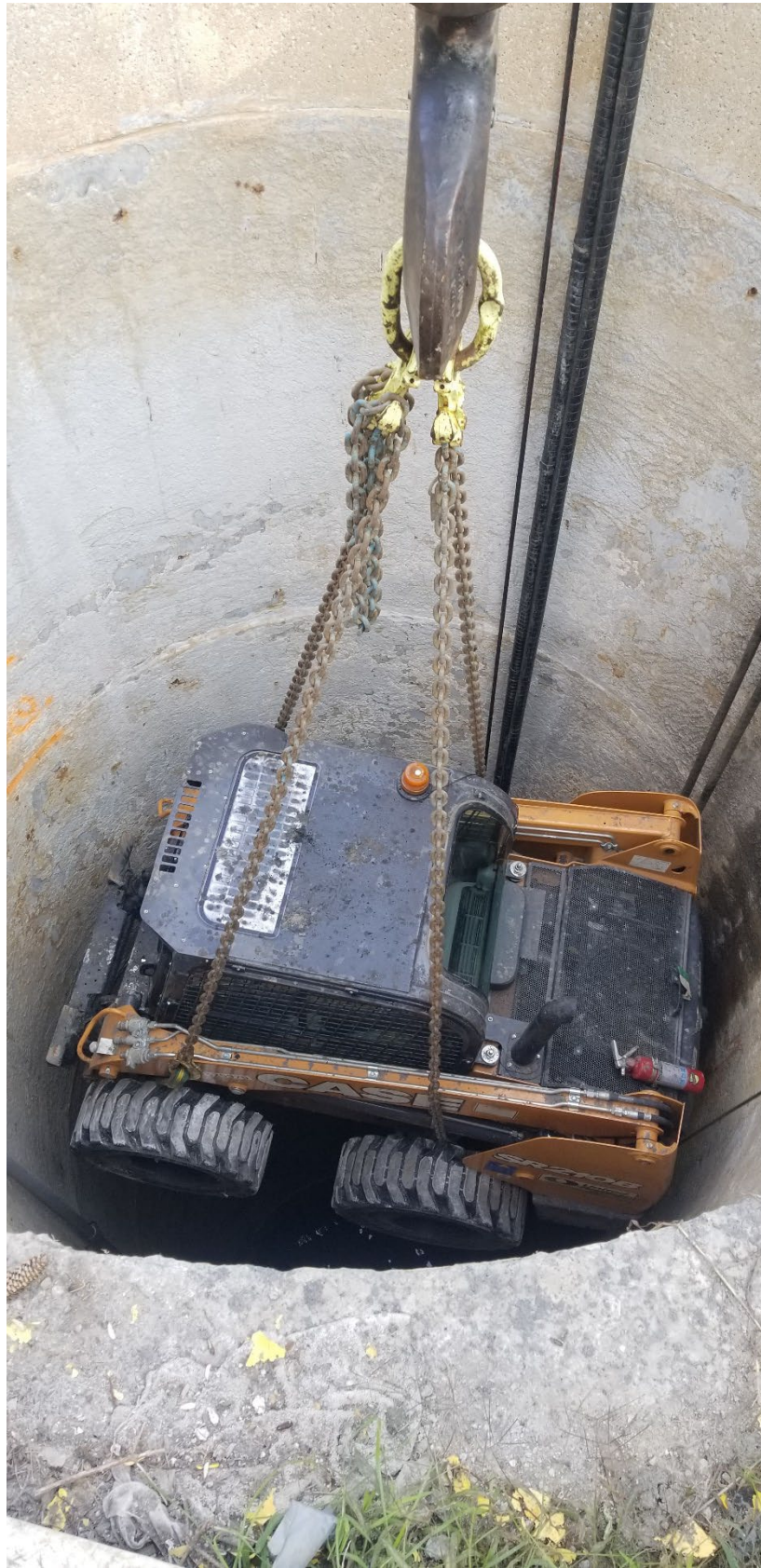
Figure 5 – Lowering in Skid-steer at MH-05
