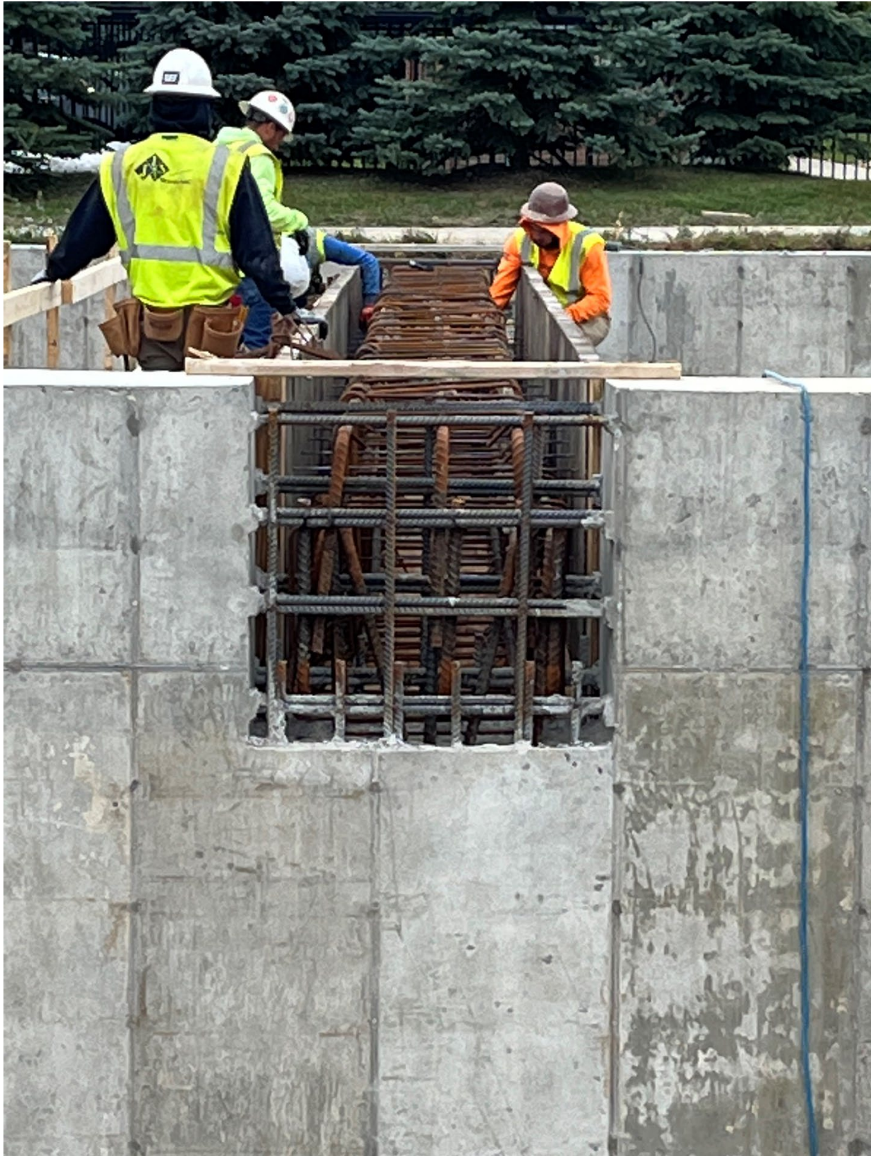
Figure 14 – Fraser Bio-Filter Roof Beam Construction
