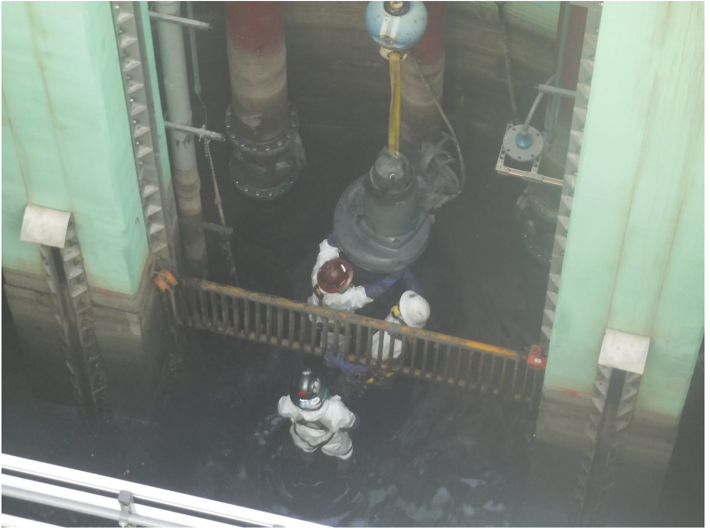
Figure 6 – ORC Performing Pump Maintenance at CS-12
