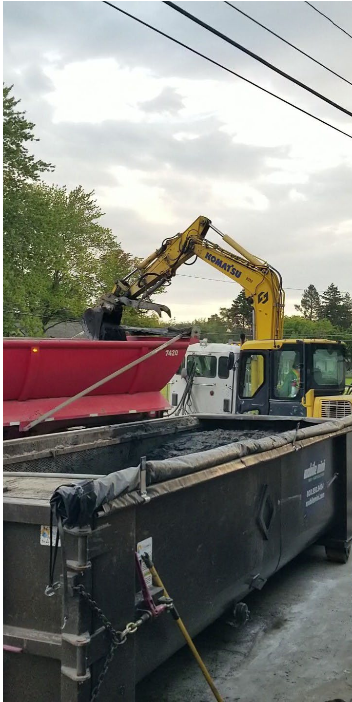
Figure 4 – Transferring Debris to Truck for Haul Off at MH-05
