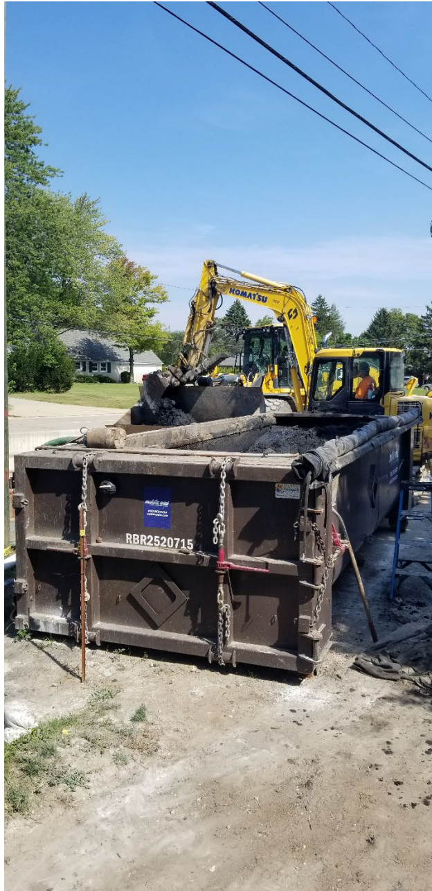
Figure 3 – Unloading Debris at MH-05
