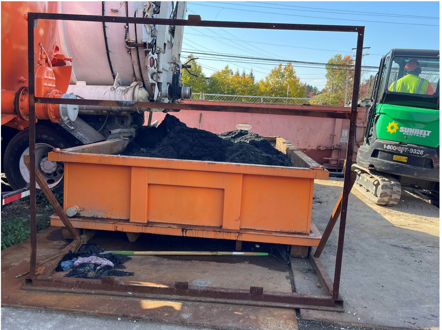
Figure 11 – RAI Curve Debris Removal
