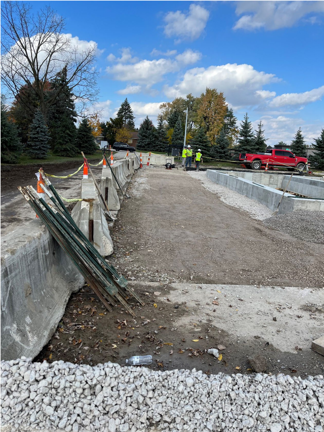
Figure 16 – Fraser Bio-Filter Backfill & Compaction
