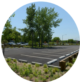
Parking areas incorporating green stormwater infrastructure
