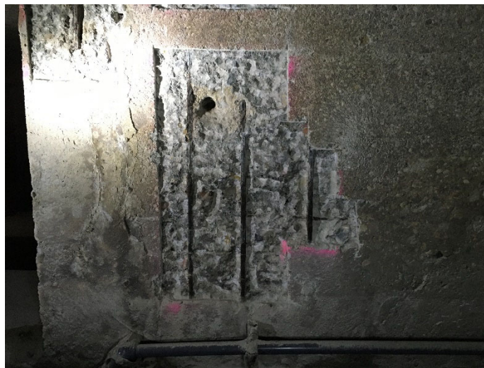
Figure 2 – Typical 9MD repair area – after demo, before patch
