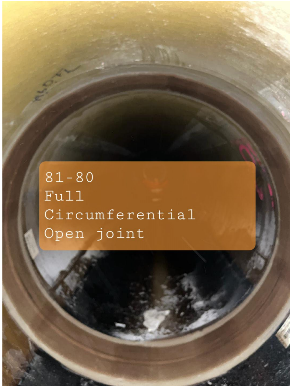
Figure 11 – HOBAS Joint Repair
