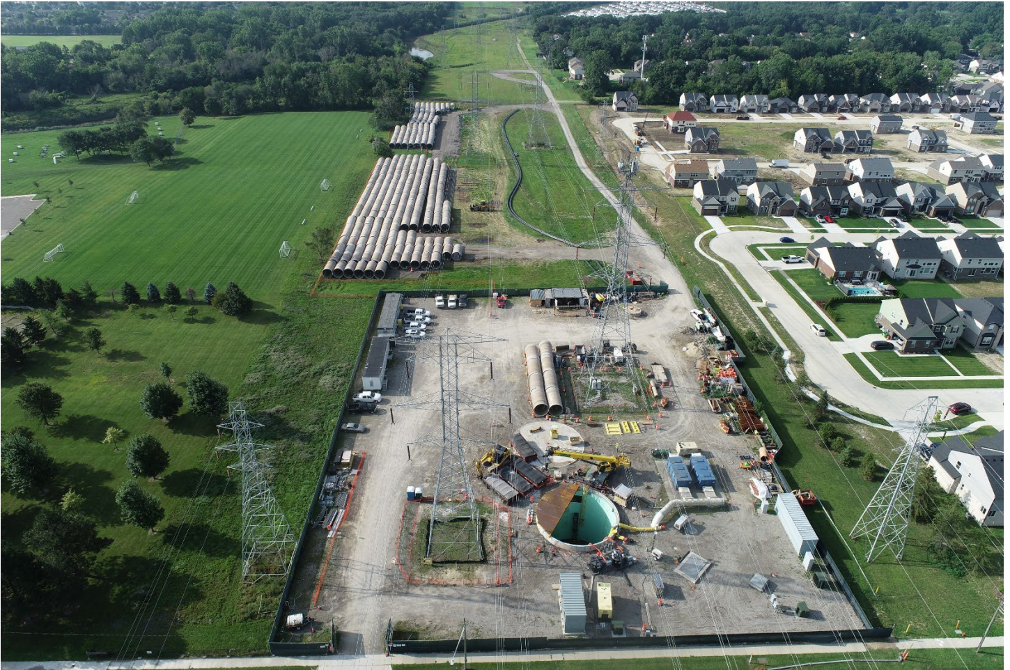
Figure 1 – CS-12 Pump Station, Construction Yard & HOBAS Storage
