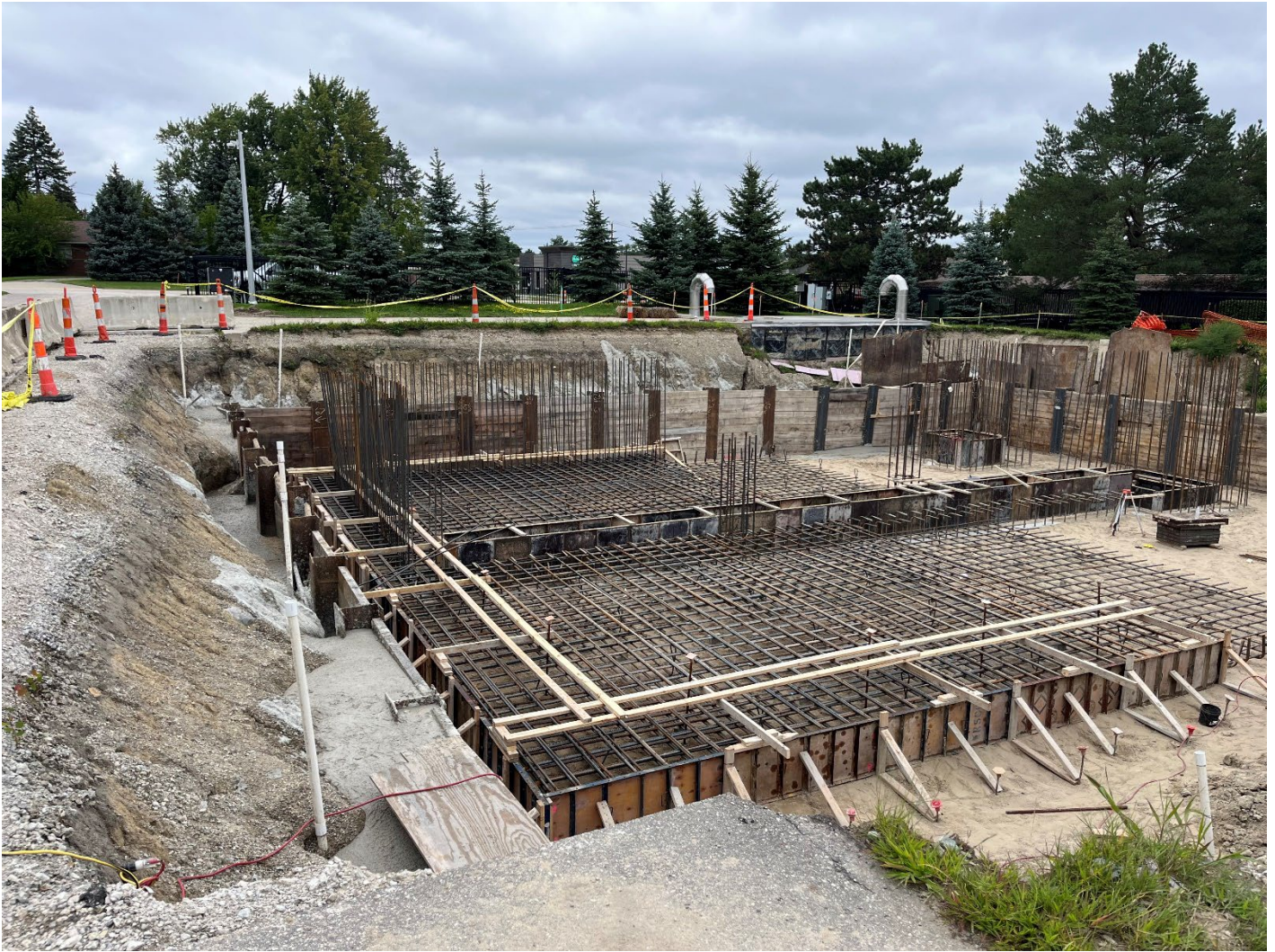
Figure 13 – Fraser Biofilter Foundation Rebar & Formwork
