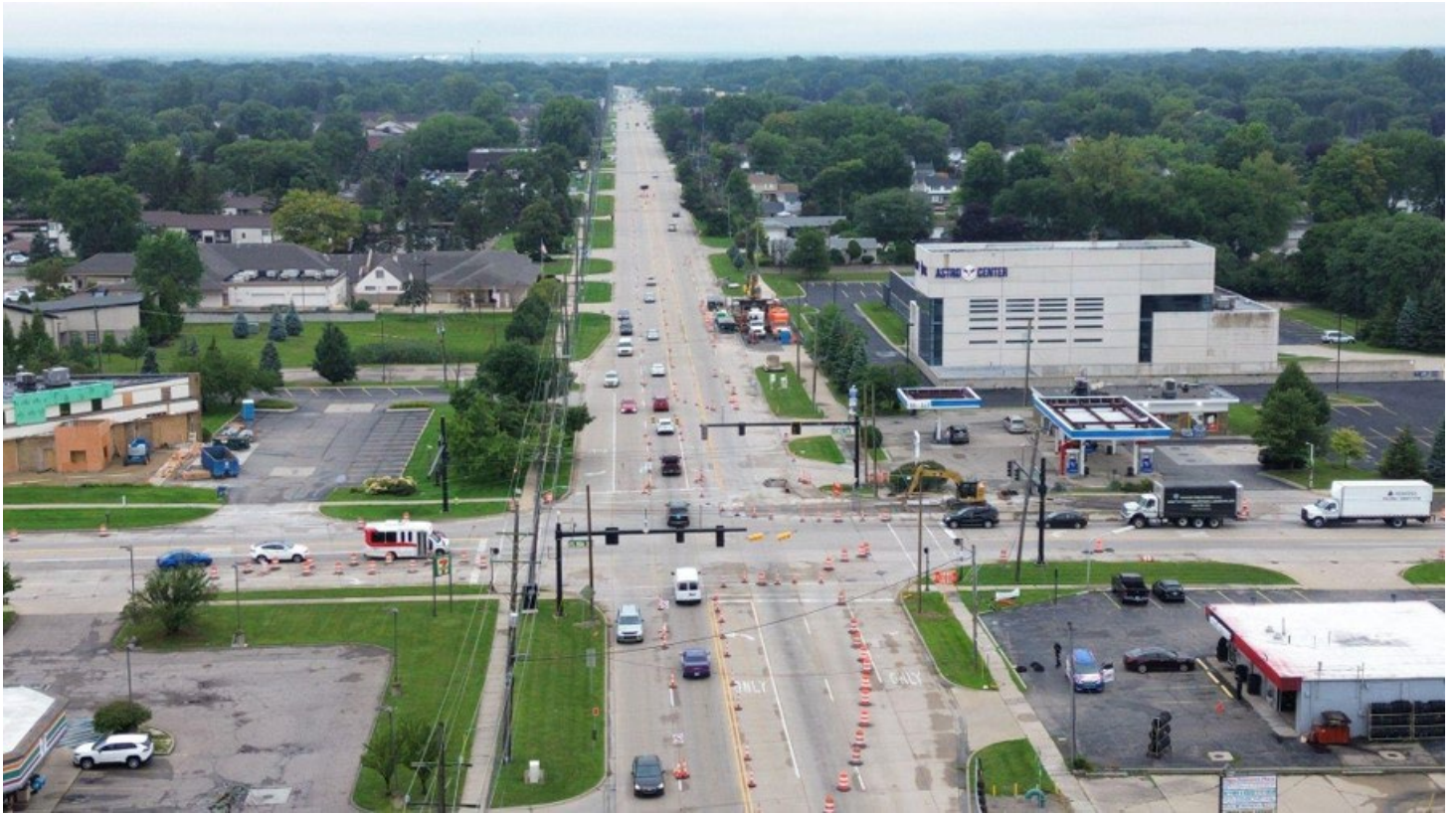
Figure 12 – Garfield Open-cut FAD Installation – Aerial View
