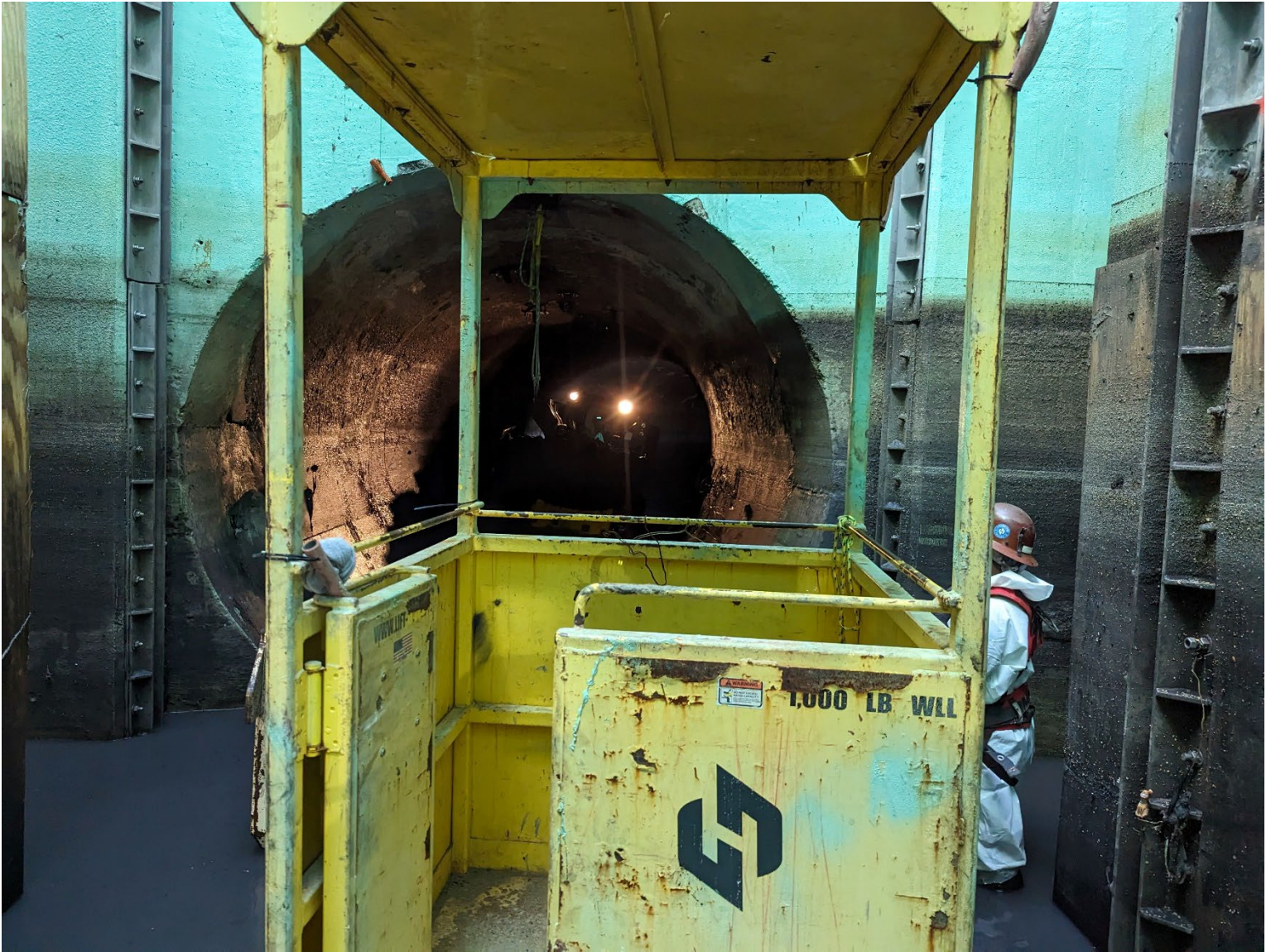
Figure 3 – Skid-Steer Returning to CS-12 during Debris Removal Operation
