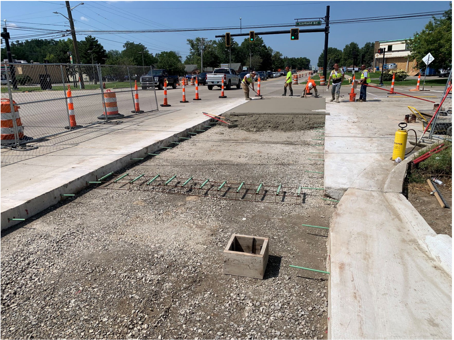
Figure 10 – Pavement Replacement at 15 Mile & Garfield after FAD Installation – Phase 1
