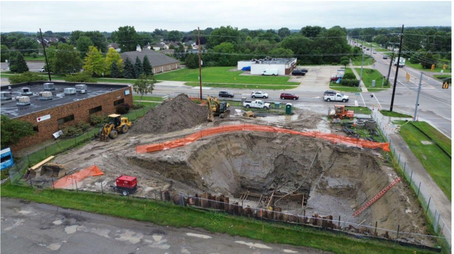
Figure 18 – Aerial View of Macomb Township Site – 21 & Garfield
