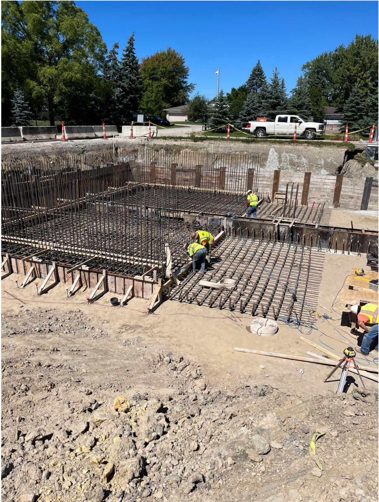
Figure 14 – Foundation Wall Rebar Installation at Fraser Site
