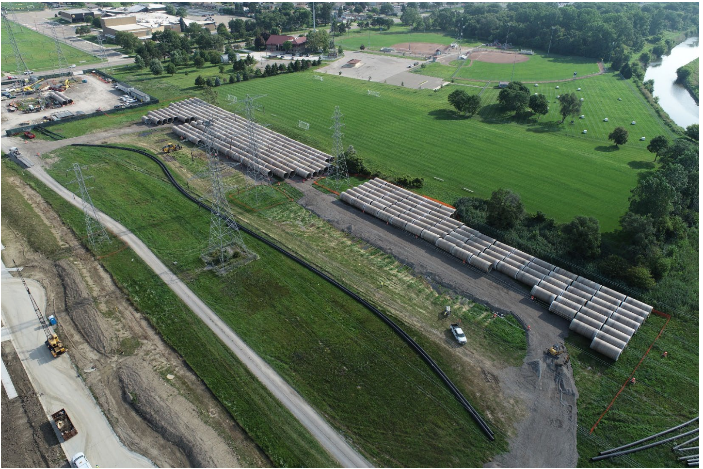
Figure 2 – HOBAS Temporary Staging in ITC Corridor
