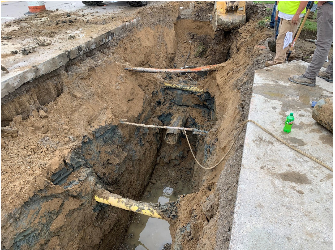
Figure 7 – Excavation for FAD Installation
