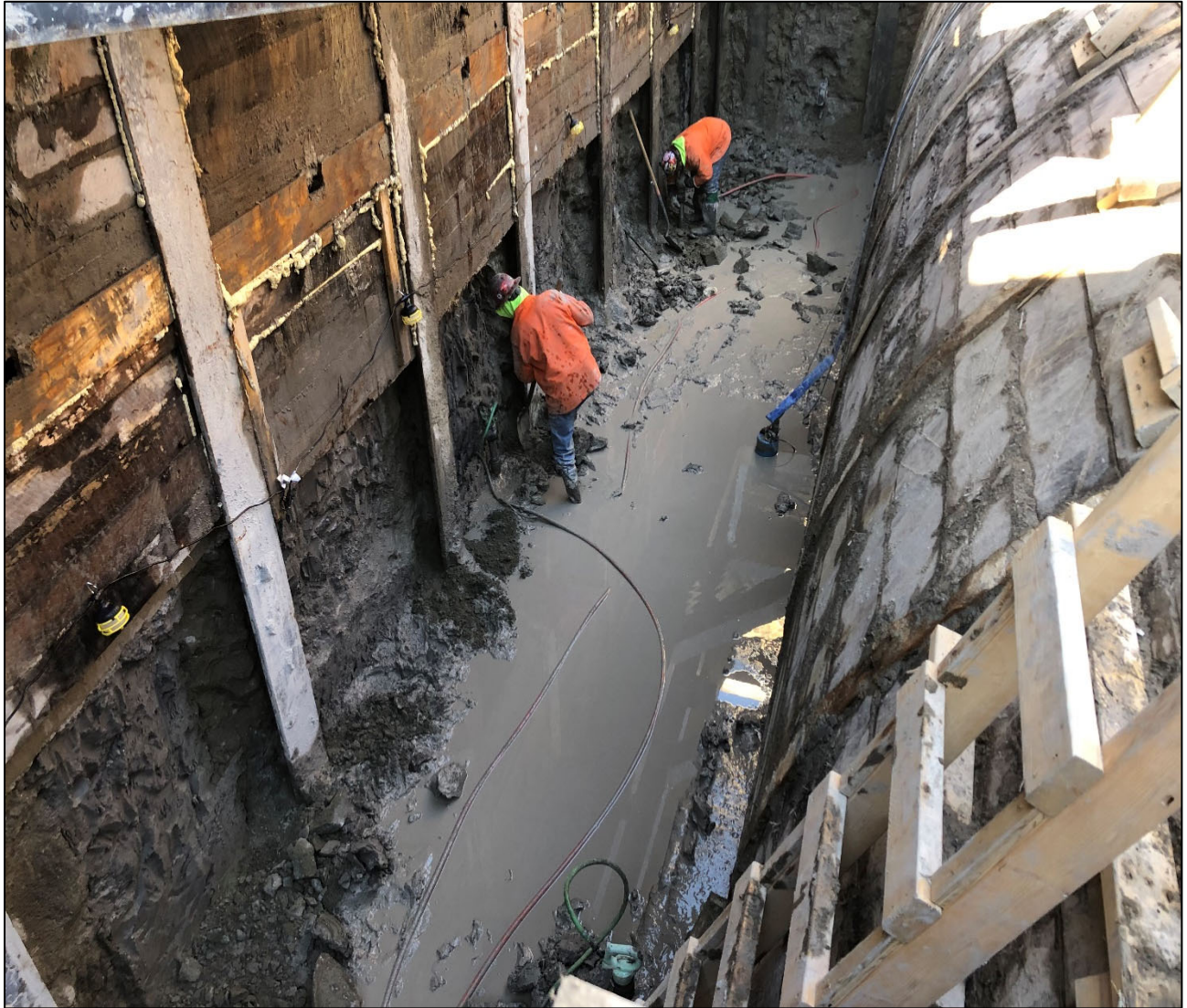
Figure 2 – Preparing to Install Lagging South Side of Tunnel
