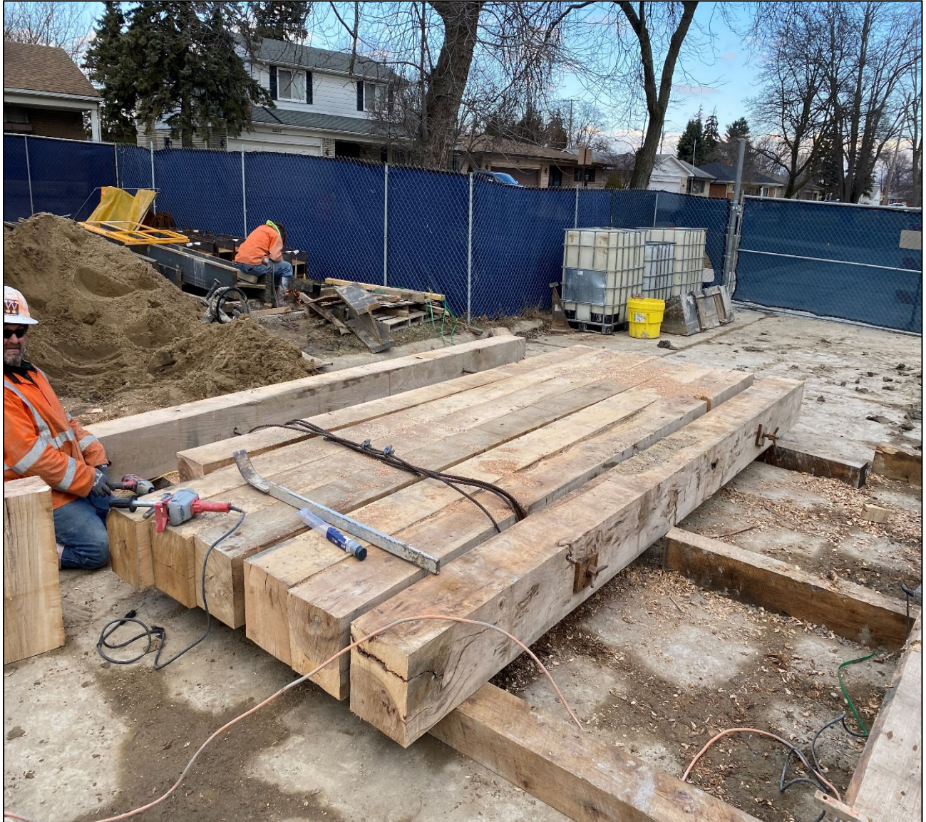
Figure 5 – 15ft Tunnel Support Timber
