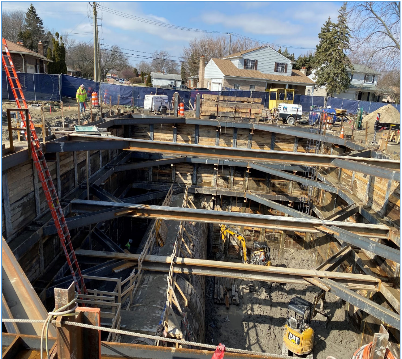
Figure 6 – Excavated Approx. 32FT Facing East
