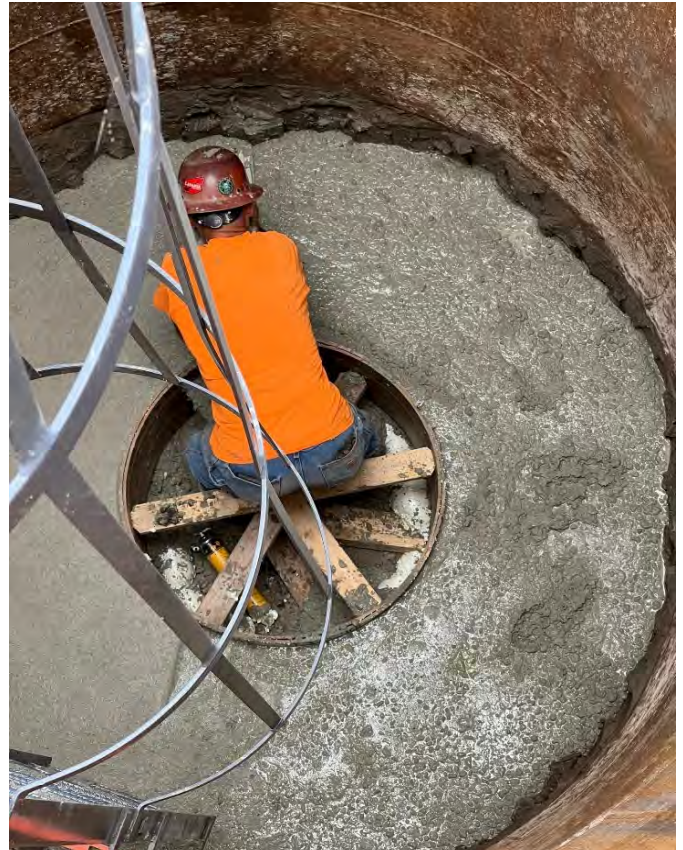
Figure 1 - Shaft to Top of 8-1/2 Relief Pipe at Gaukler & Kelly Sites; Concrete Collar Placements
