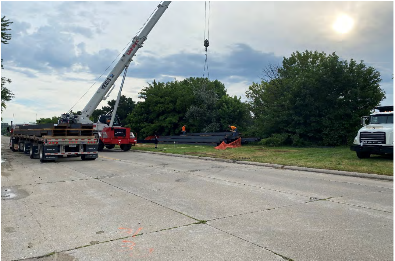
Figure 4 – Unloading Delivery of 40ft Steel Piers
