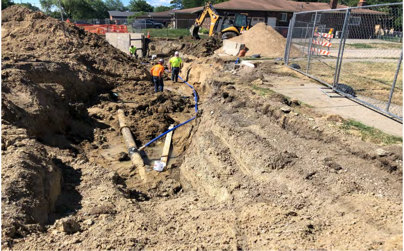
Figure 2 – Water Main Bypass at Beaconsfield and Oak
