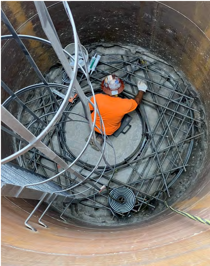
Figure 1 - Shaft to Top of 8-1/2 Relief Pipe at Gaukler & Kelly Sites; Concrete Collar Placements
