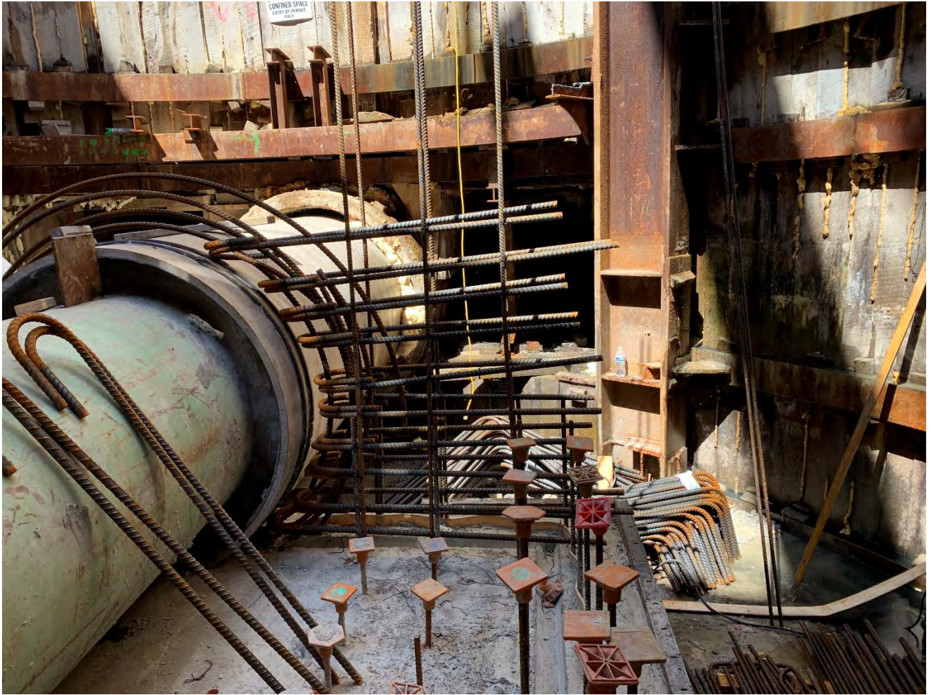
Figure 10 - CS-13 Wall Re-steel Installation
