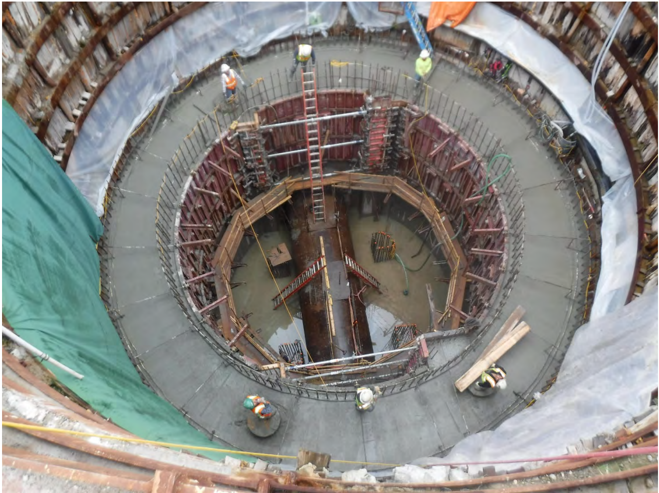
Figure 1 – CS-12 Wall Lift #2
