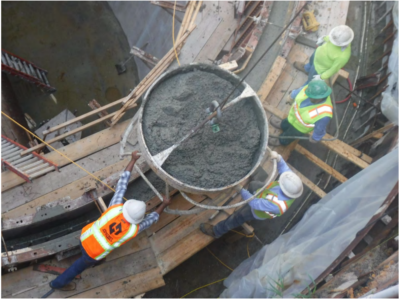
Figure 2 – CS-12 Flume Wall Concrete Placement
