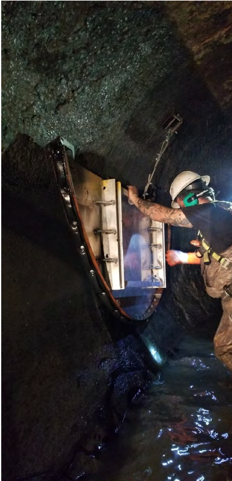
Figure 3 – Aluminum Bulkhead Storage Position
