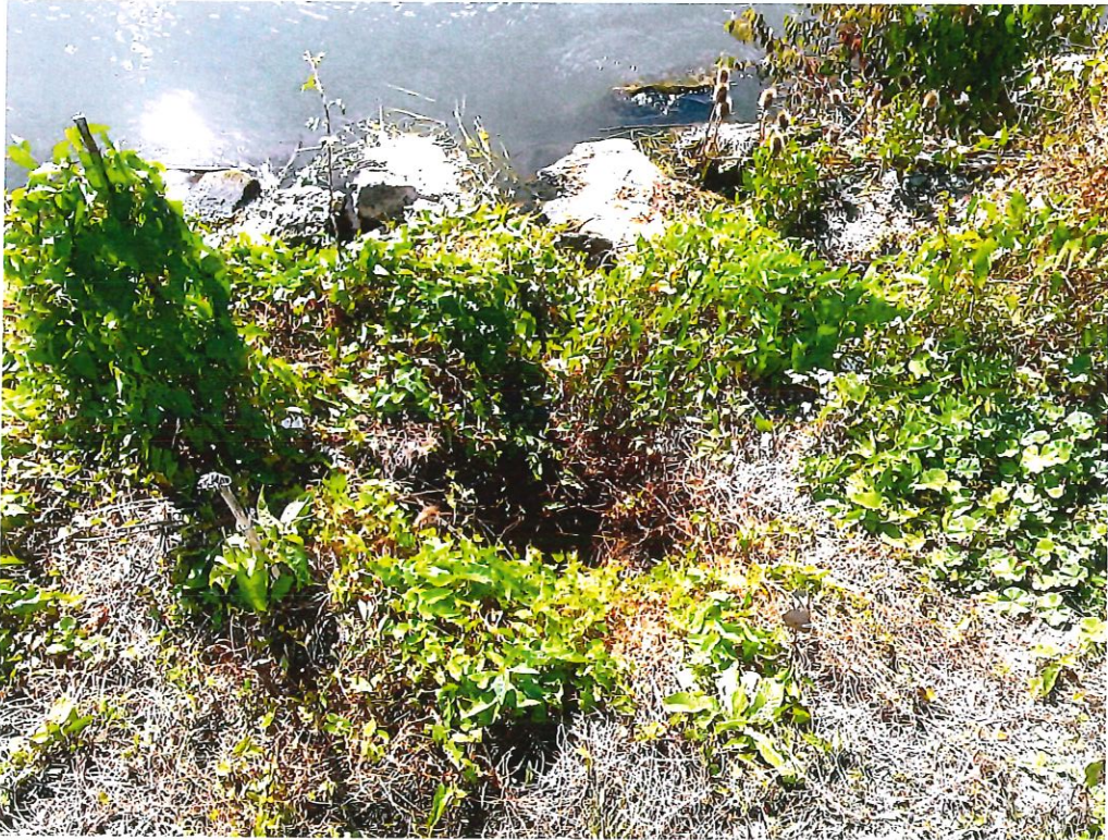
Photo 11: Area of plantings/ shore stabilization. Erosion control fabric and soil appear to have been placed over riprap.
