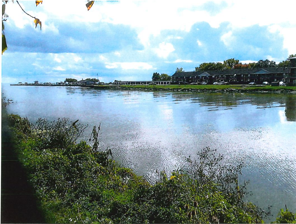
Photo 9: Right bank of channel near Lake St. Clair. Note erosion.
