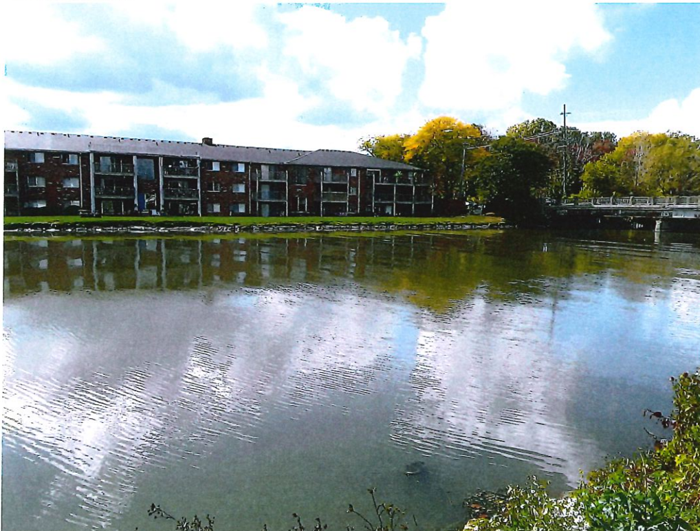
Photo 8: Right bank of channel, looking toward Jefferson Ave. Note erosion.
