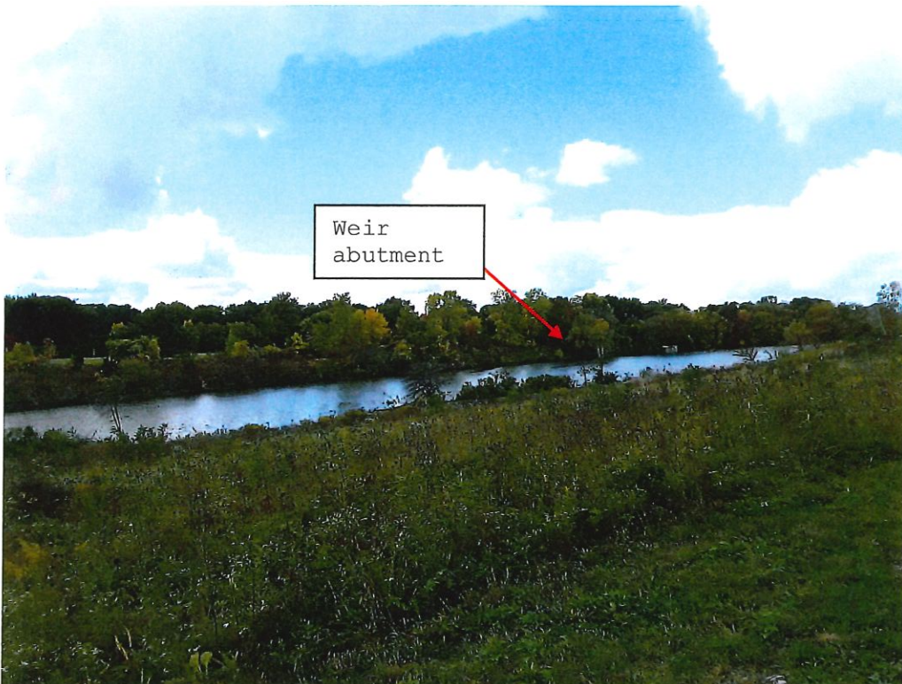
Photo 2: Cutoff channel looking upstream at weir from north (left) bank.
