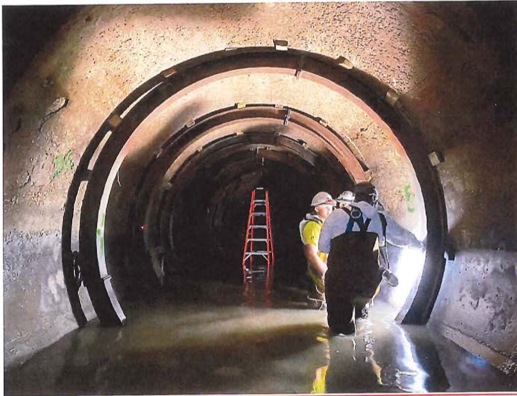
Figure 7 - Relocation of Steel Ribs
