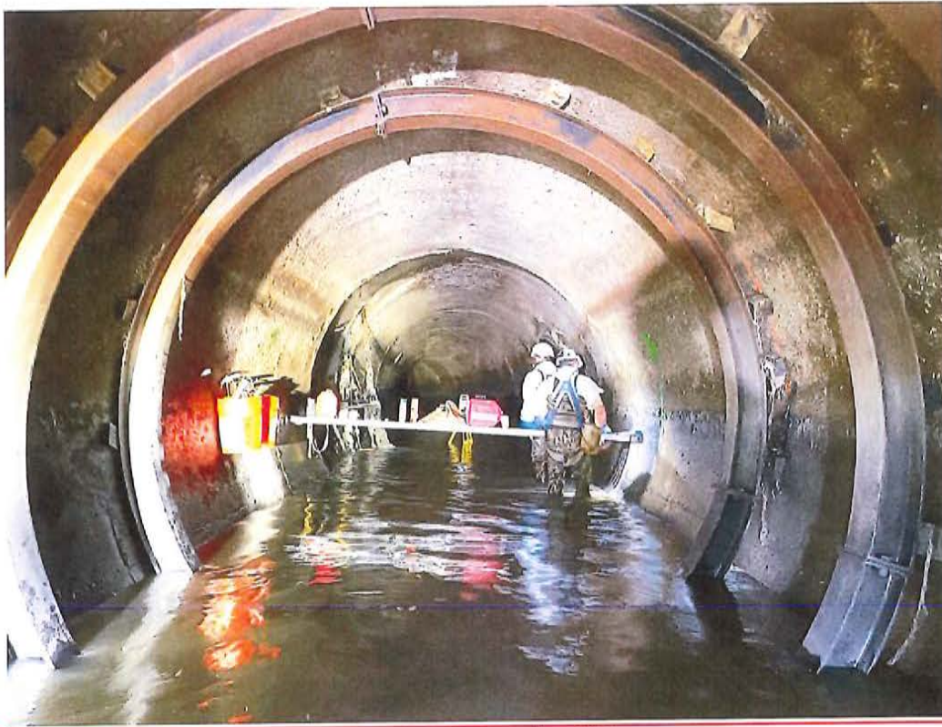
Figure 6 - Relocation of Steel Ribs
