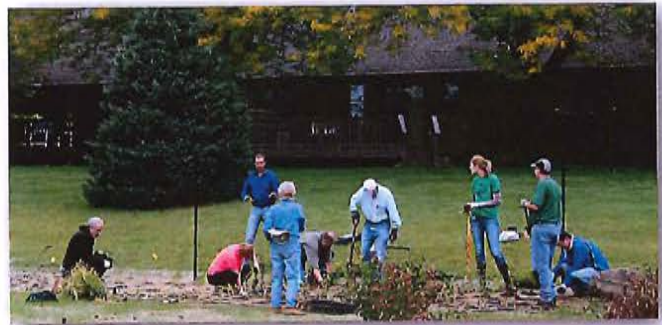
Tetra Tech team constructing green infrastructure in the City of Detroit.
