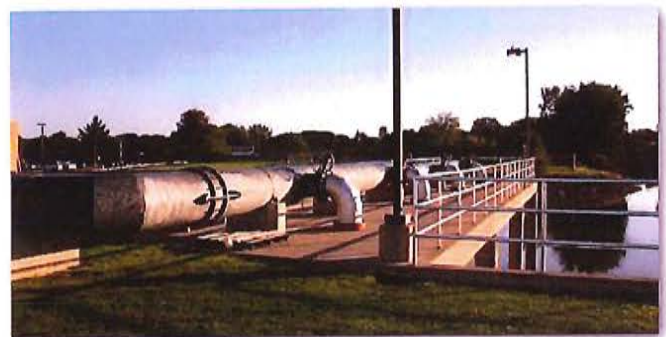
Milk River CSO Retention Basin
