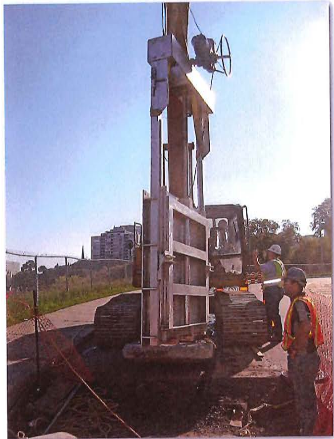
Tetra Tech team installing a sluice gate
