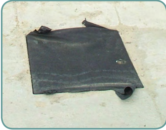
Good application of an inlet grate wrapped with a geotextile.
