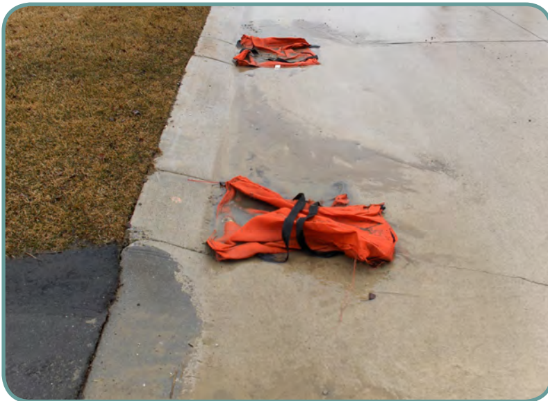
Protect stormwater inlets with commercial dike products or site-fabricated ponding berms made of rock, wire, or other material. If the inlet filter system is causing ponding in the roadway, an inlet filter bag or other low-profile product may be beneficial. For best results, sediment should be retained on the landscaped areas and not discharged into roadways or parking lots. This photo shows an example of commercially available inlet filter bags that are properly installed and effectively protecting two inlets.
