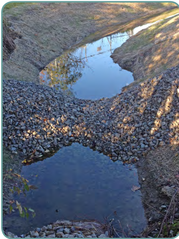
Small, temporary sediment traps intercept and detain construction site runoff so soil particles can settle out. Designing traps and basins with long flow paths between the inlet and outlet also helps to increase sediment removal efficiency by extending the detention time. Where space restrictions prevent long basin designs, barriers placed in the basin can lengthen detention times by creating a serpentine flow path between the inlet and outlet. This photo shows an example of a sediment trap in a drainage ditch with a check dam.
