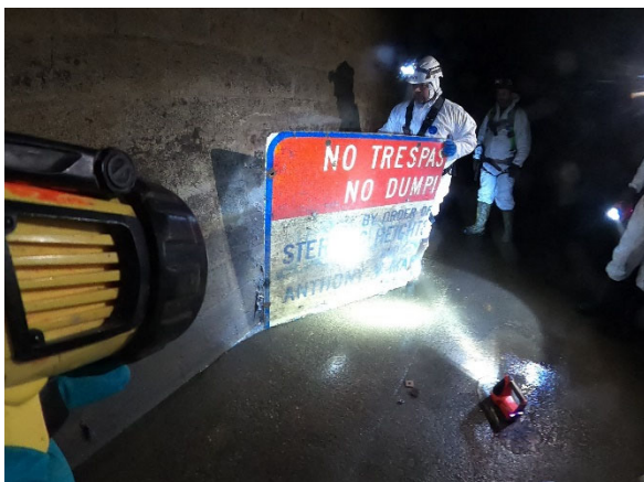
Figure 1 – Crews re-configuring temporary stoplogs
