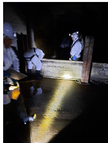
Figure 2 – Crews re-configuring temporary stoplogs
