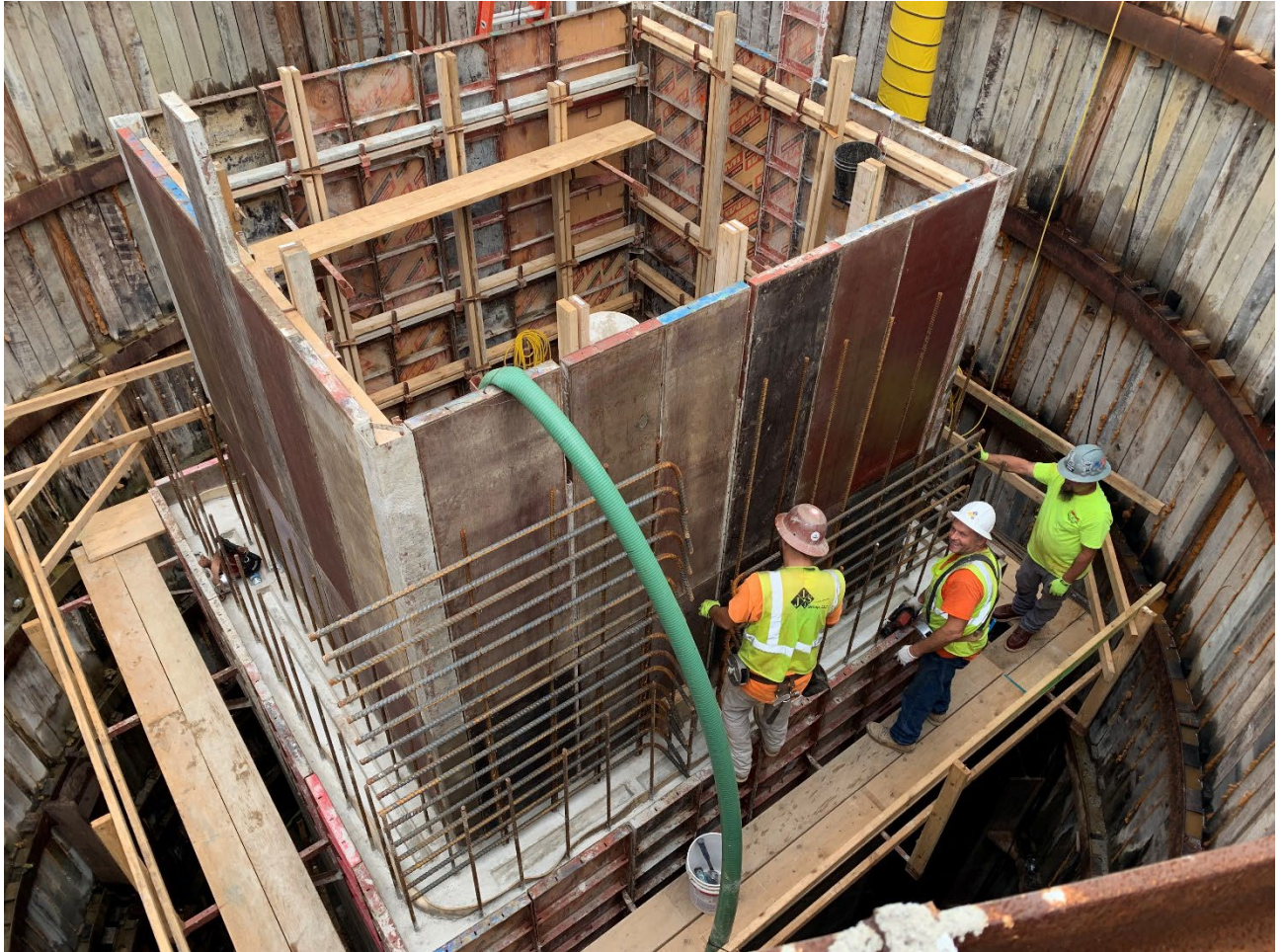
Figure 9 - Installing Rebar for Structure Walls
