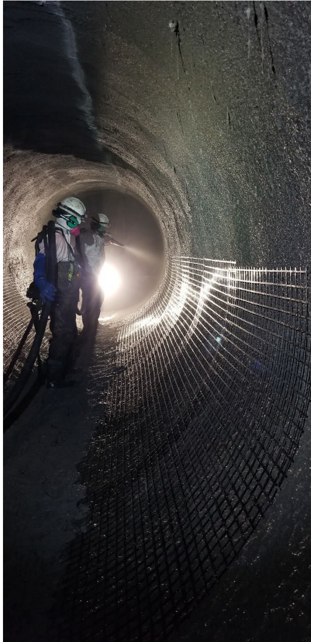
Figure 1 – Geo-Polymer Spray Lining in PCI-37
