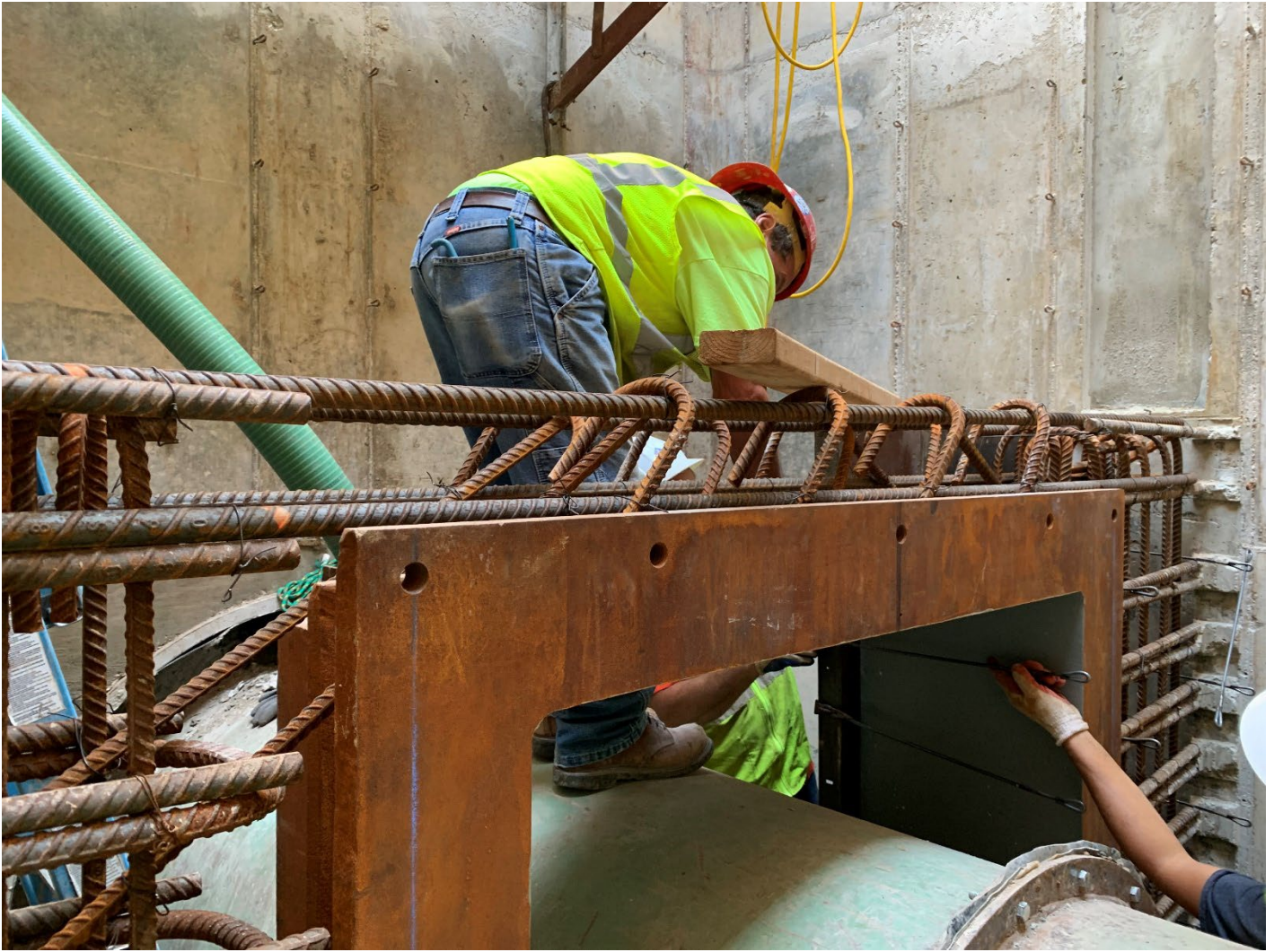
Figure 6 - Installing Rebar around Thimble
