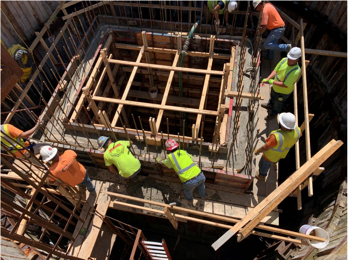
Figure 8 - Concrete Placement for Structure Walls
