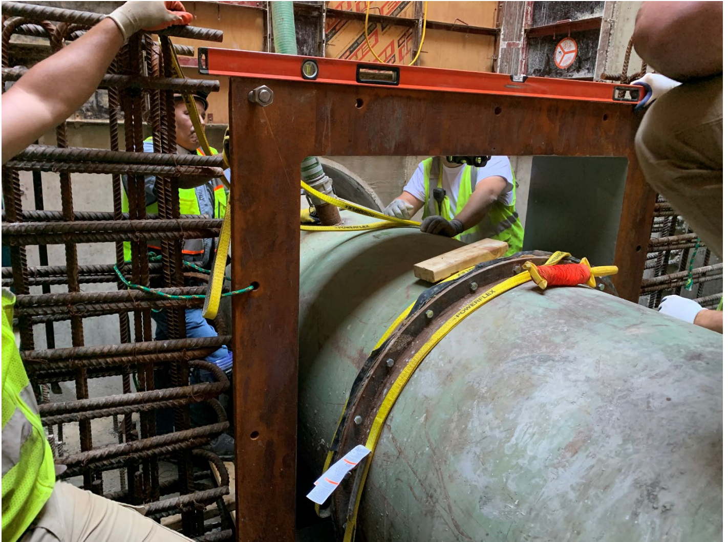
Figure 7 - Verifying the Thimble is Level
