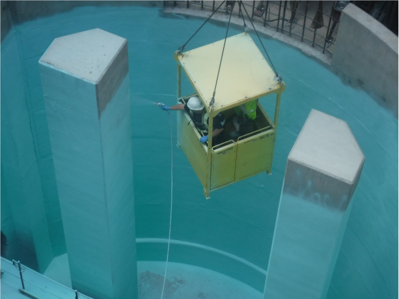
Figure 3 – CS-12 Protective Epoxy Coating Application
