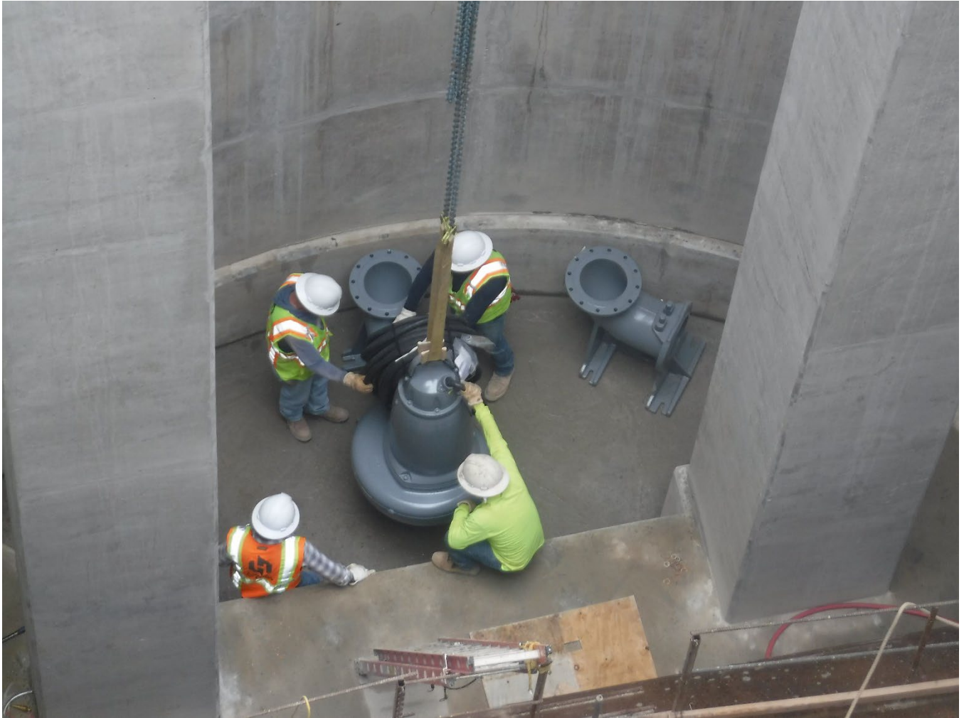
Figure 4 – Dry-fitting the CS-12 Pumps Prior to Application of Protective Epoxy Coating
