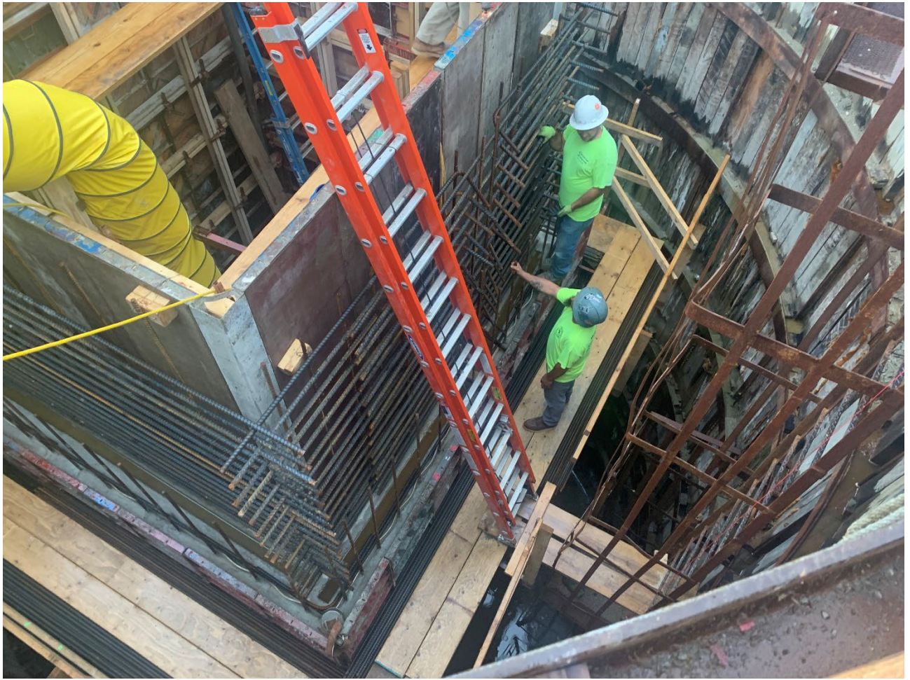
Figure 10 - Rebar Installation for Structure Walls
