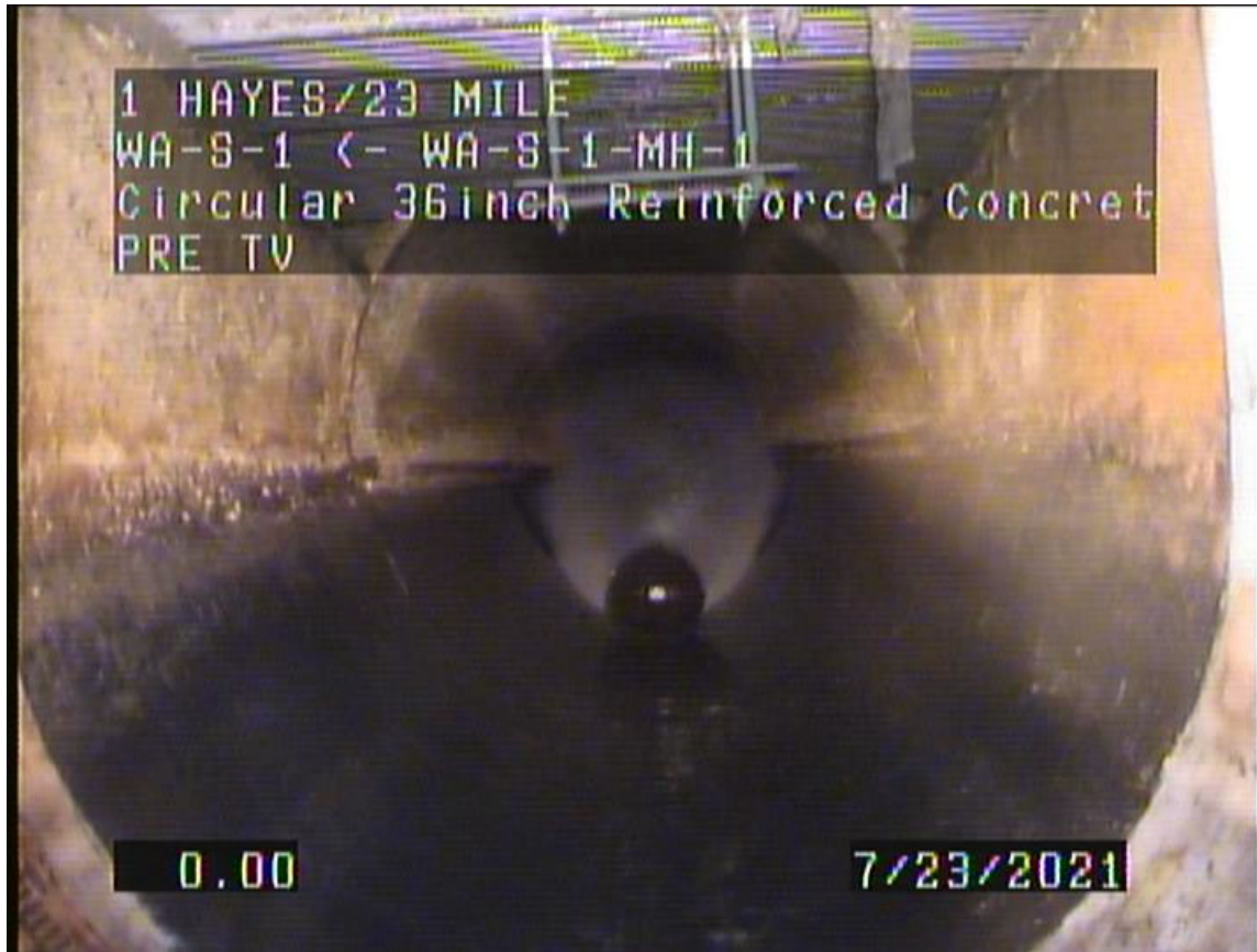
Figure 6 - WA-S-1 Connecting Sewer Initial CCTV Inspection
