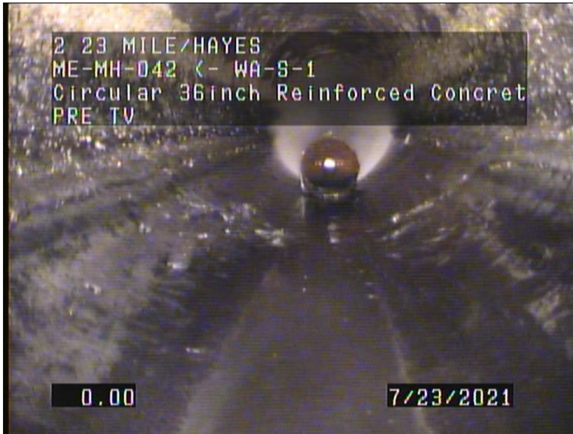
Figure 7 - WA-S-1 Connecting Sewer Initial CCTV Inspection
