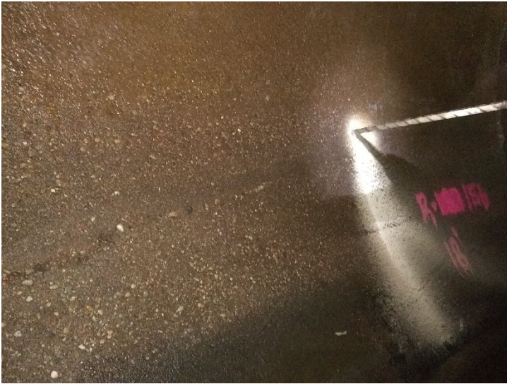
Figure 3 - Drilling for Grout Port Installation
