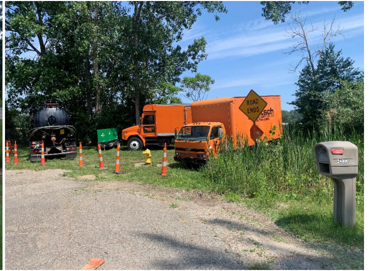
Figure 4 - Grouting Rigs at LSI-MH006 at Ballard Street
