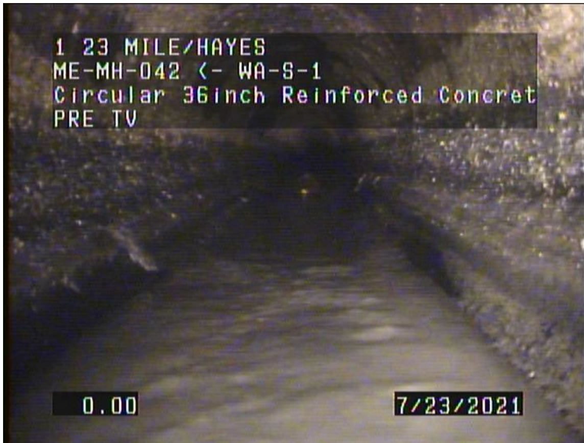
Figure 8 - WA-S-1 Connecting Sewer Initial CCTV Inspection
