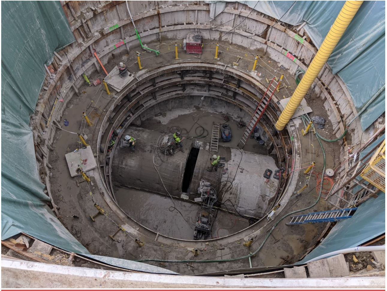
Figure 4 - First Section of Interceptor Removed
