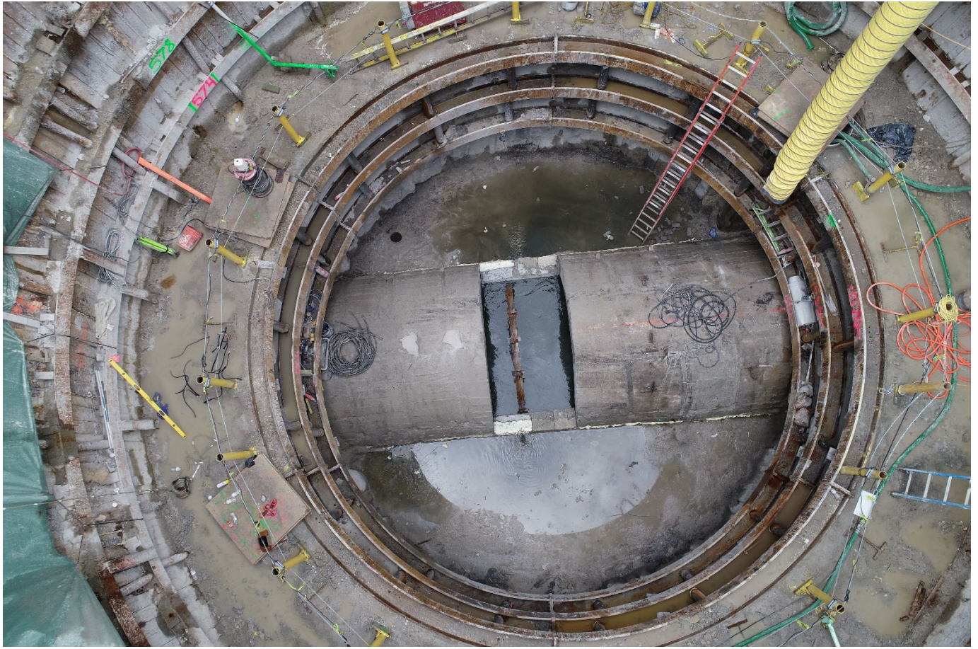
Figure 5 - Interceptor Demolition
