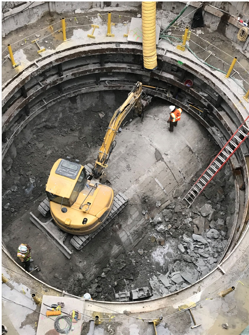
Figure 1 – Excavating & Exposing the Interceptor
