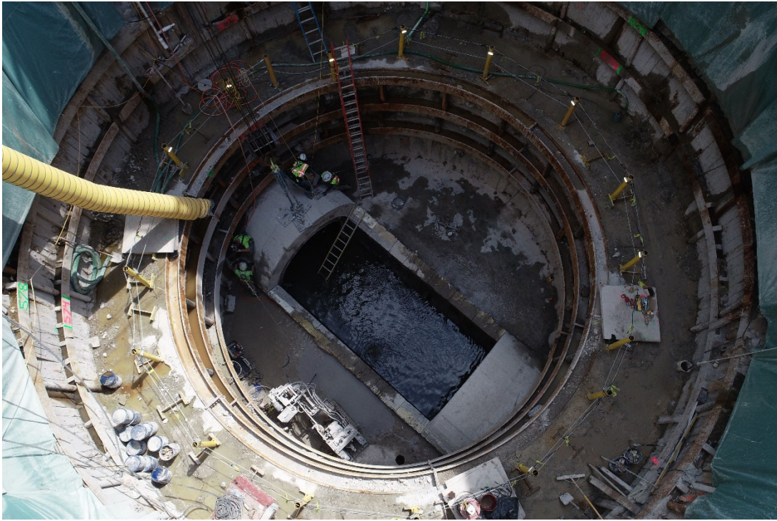
Figure 6 - Interceptor Demolition
