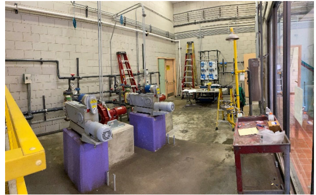
Figure 1b – Pump Room piping – After pipe installation
