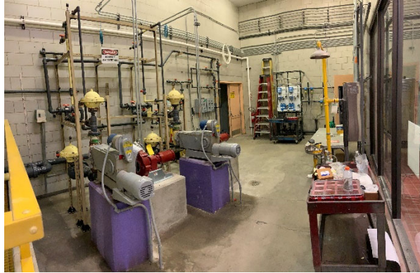
Figure 1a – Pump Room piping – Before pipe demolition
