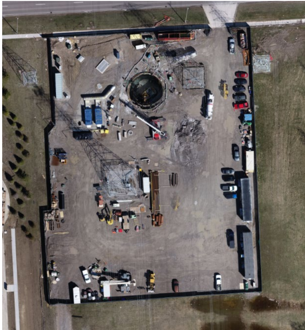
Figure 1 – April 2021 Site View
