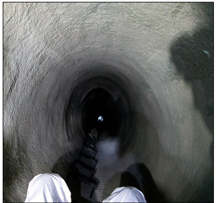
A before-and-after look at a drop shaft in Harrison Township that underwent spray lining to preserve the sewer.
