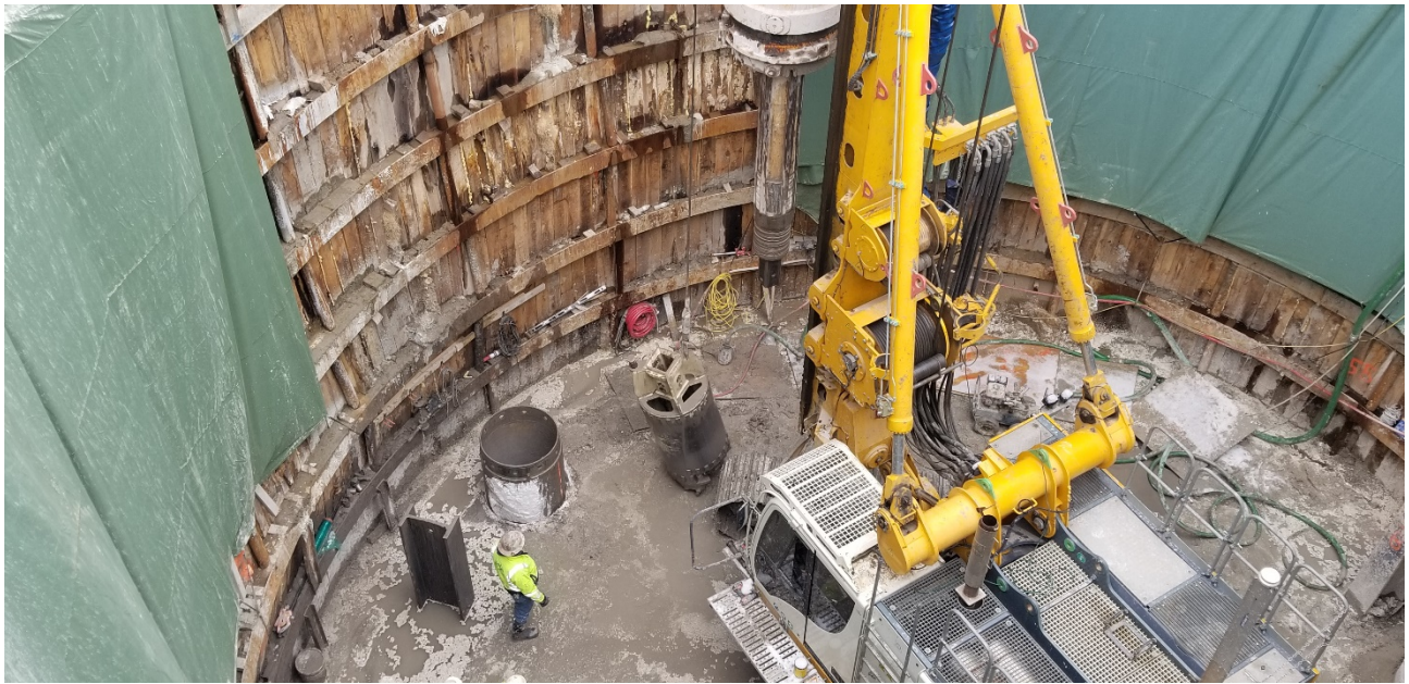
Figure 3 – Drilling Rig Head
