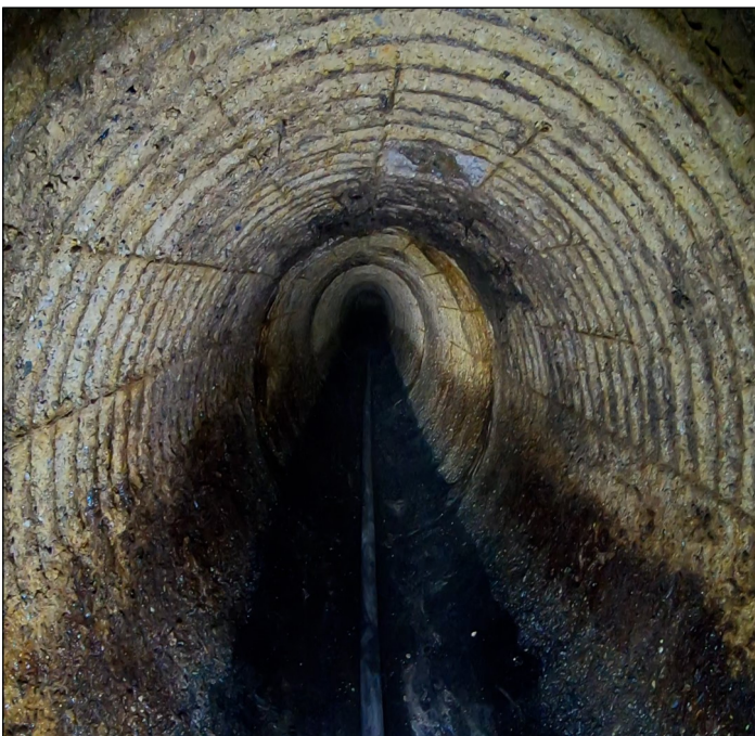
A before-and-after look at a drop shaft in Harrison Township that underwent spray lining to preserve the sewer.
