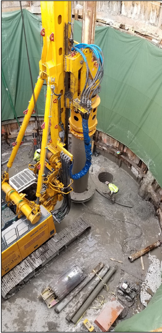
Figure 6 - Secant Pile Drilling Operation
