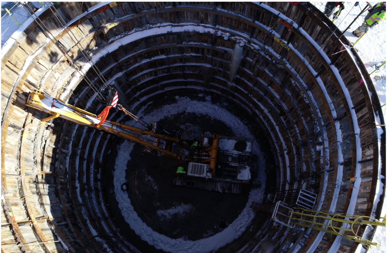
Figure 4 - Assembly of Secant Pile Drilling Rig
