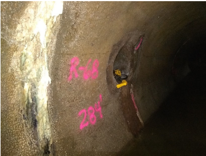
Figure 10 - Infiltration
