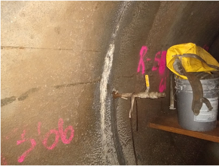
Figure 12 - Grout Port at Infiltration
