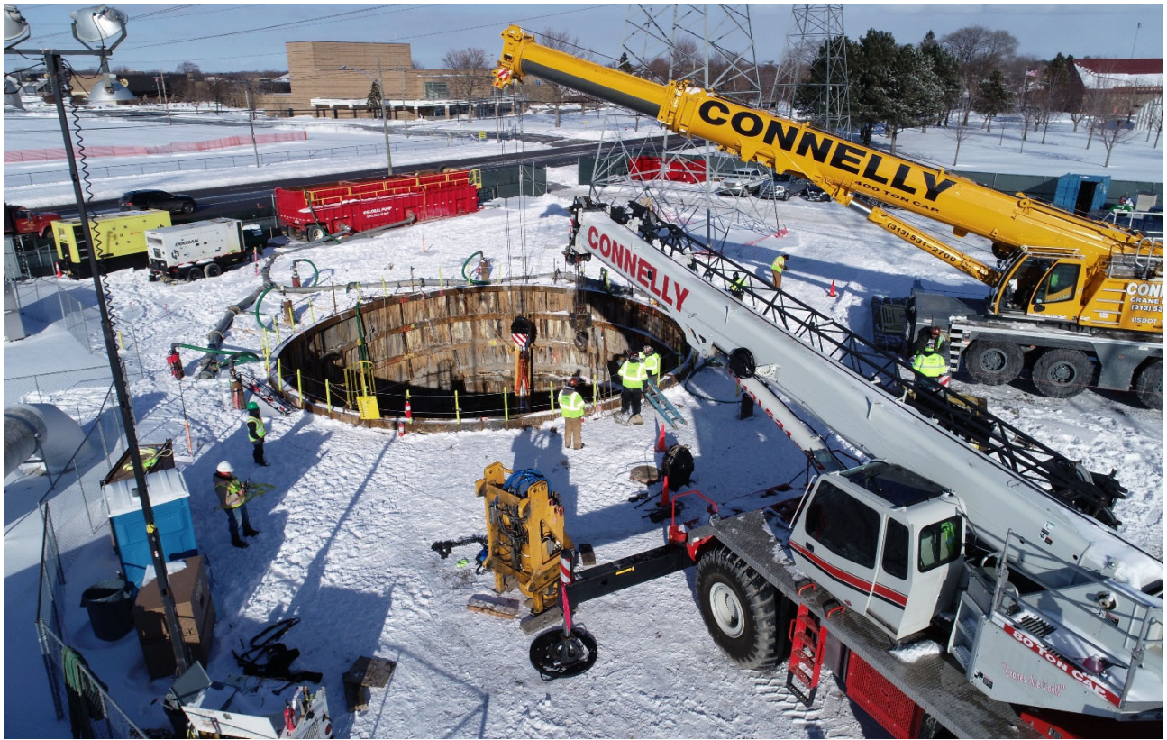
Figure 3 - Assembly of Secant Pile Drilling Rig
