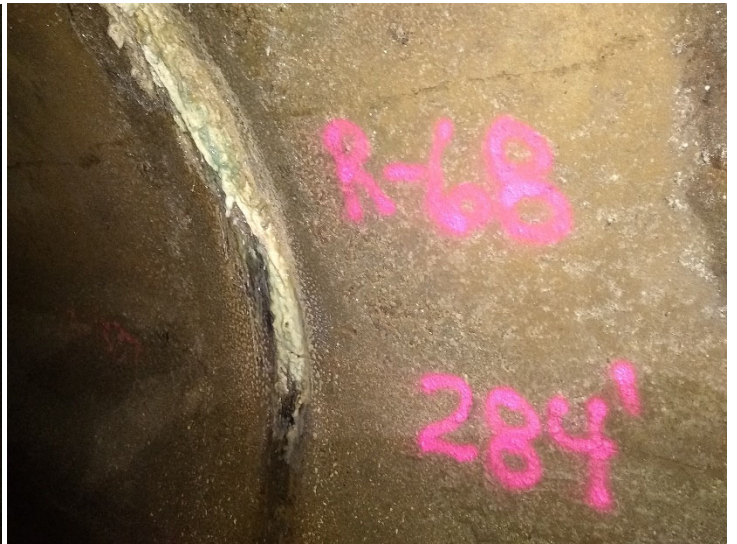
Figure 9 - Infiltration
