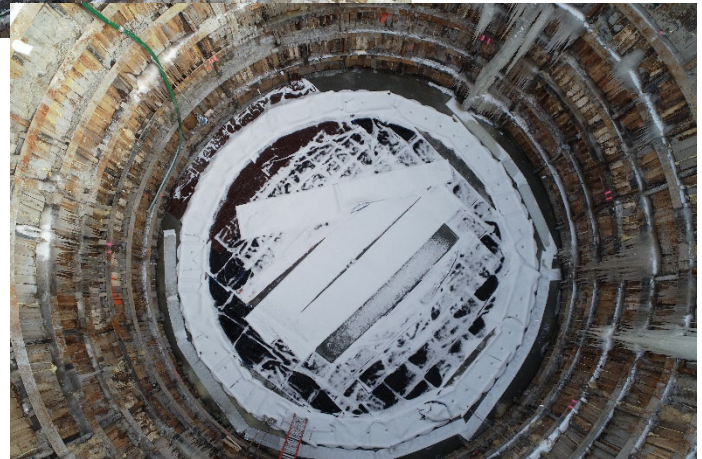
Figure 2 - Construction of Secant Pile Drilling Template
