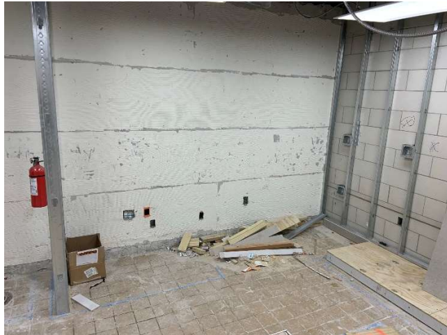
Figure 6 – Demo and partial new construction of East Building lab
