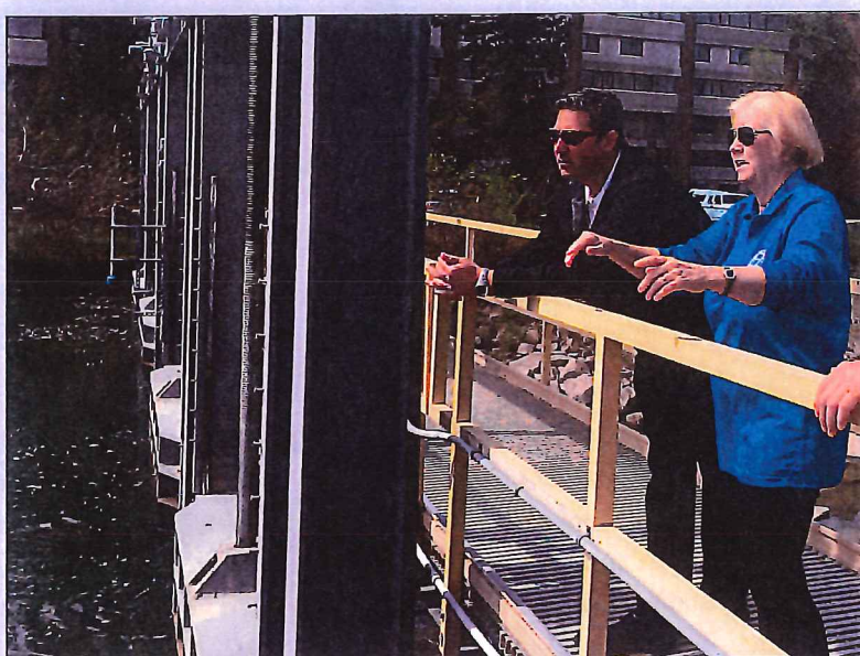
Public Works Commissioner Candice S. Miller and County Commissioner Rob Leonetti at the Chapaton Retention Basin in St. Clair Shores.
